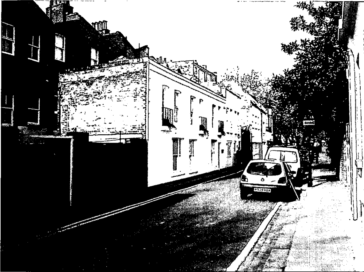
View of property before works
