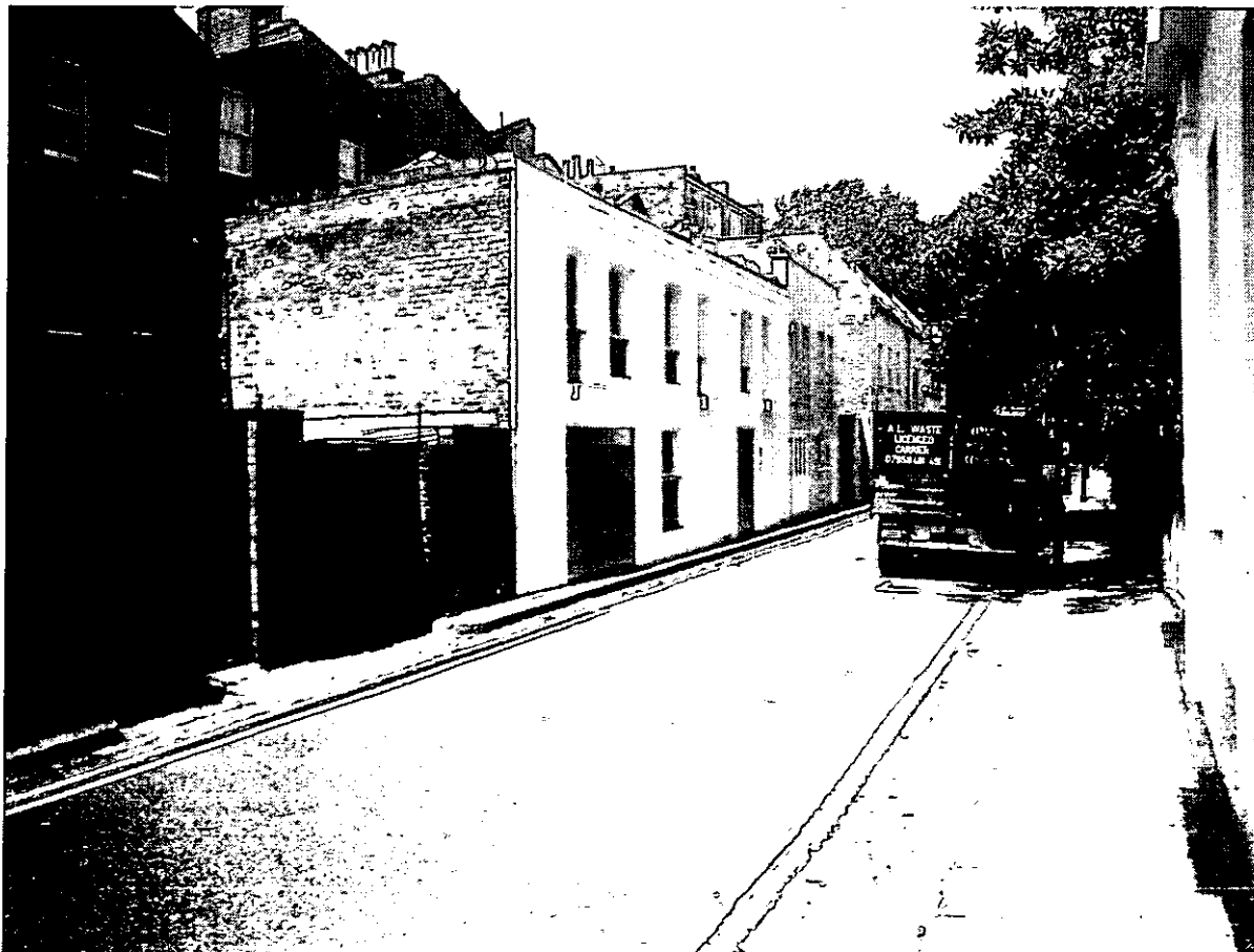
View of property after works
