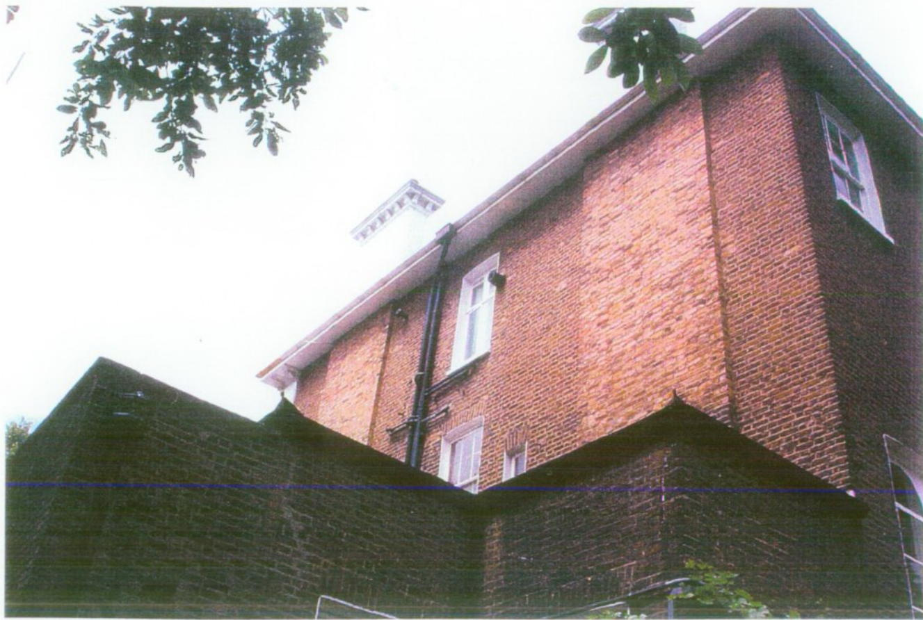
View of Side of No. 10 Of Upper Floors
