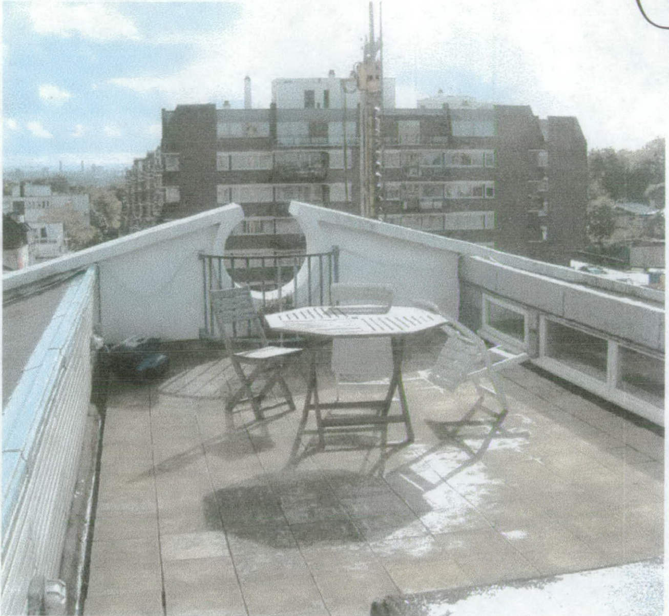
25 CAMPDEN HILL GARDENS - VIEW ON ROOF TERRACE EXISTING FACING SOUTH
