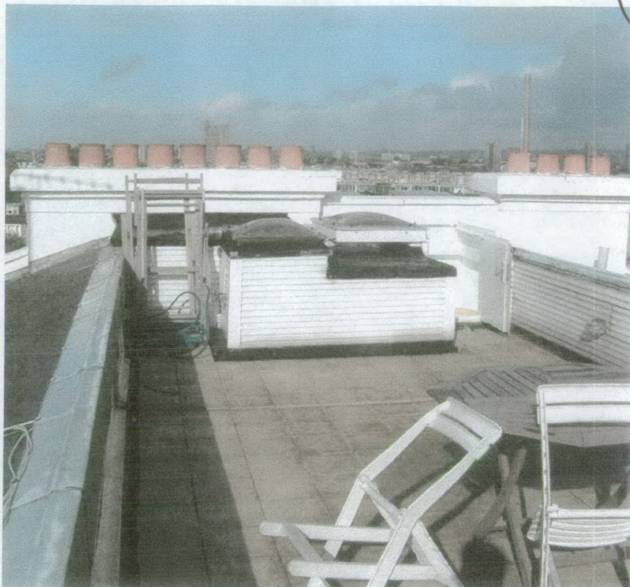
25 CAMPDEN HILL GARDENS - VIEW ON ROOF TERRACE EXISTING FACING NORTH
