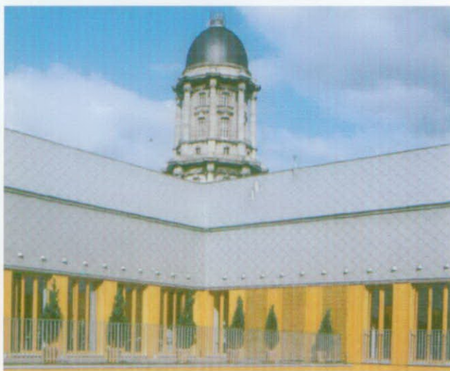
Traditional examples of zinc sheet roofing
