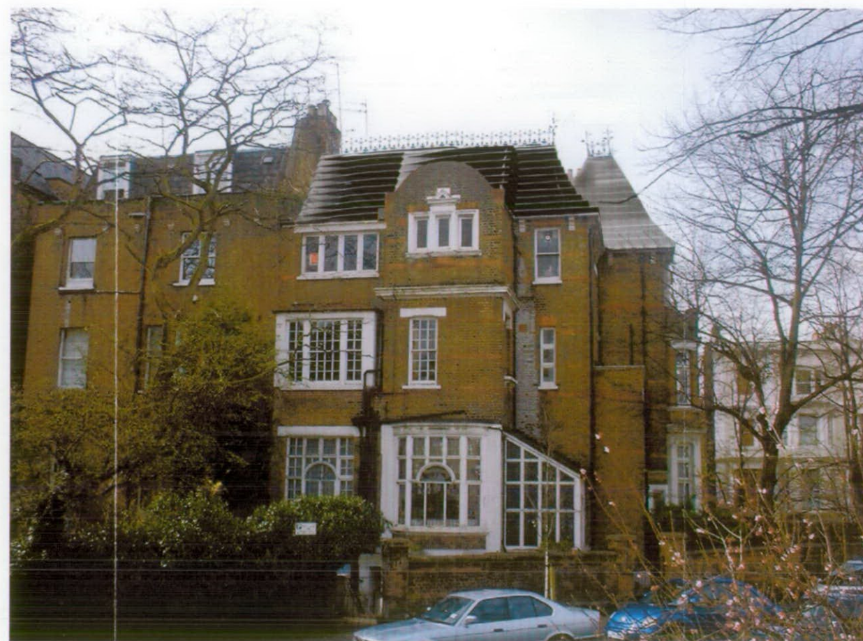
View from Addison Crescent Looking South
