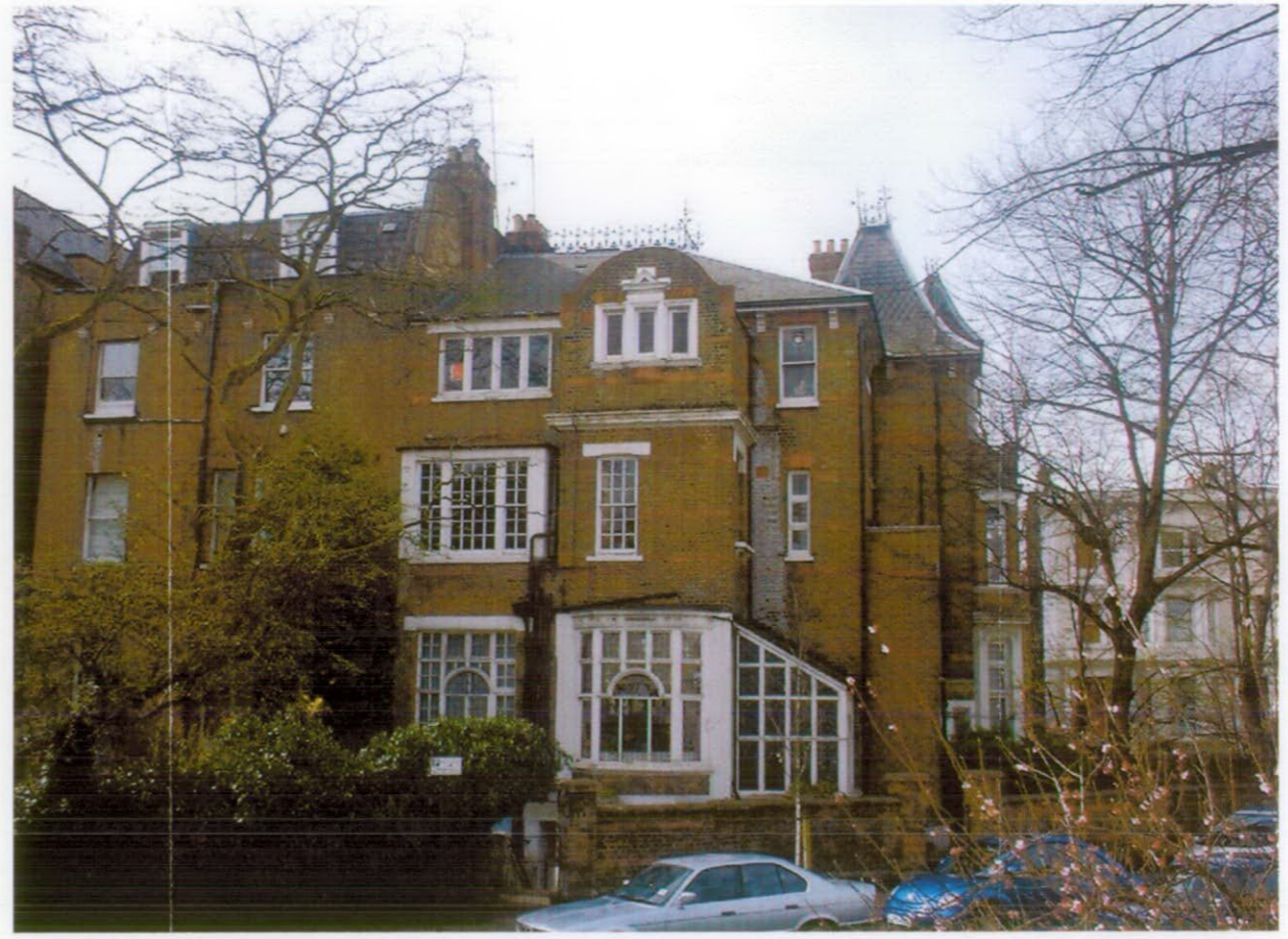
View from Addison Crescent Looking South
