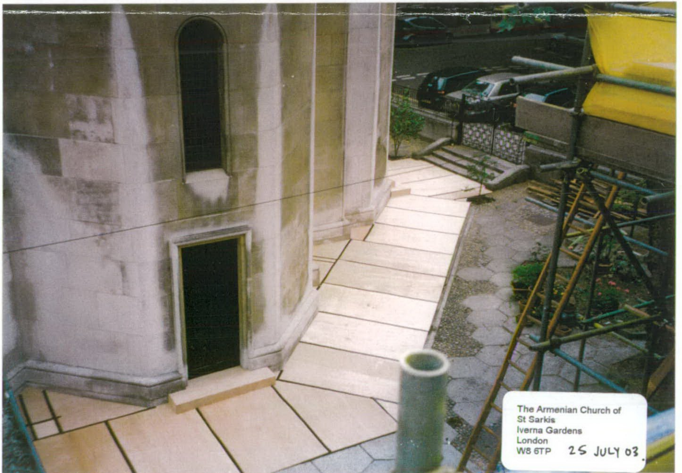
PLYWOOD PROTECTION TO ORIGINAL PORTLAND STONE PAVING & STEPS. SCAFFOLDING BY STONEWEST TO COMMENCE
