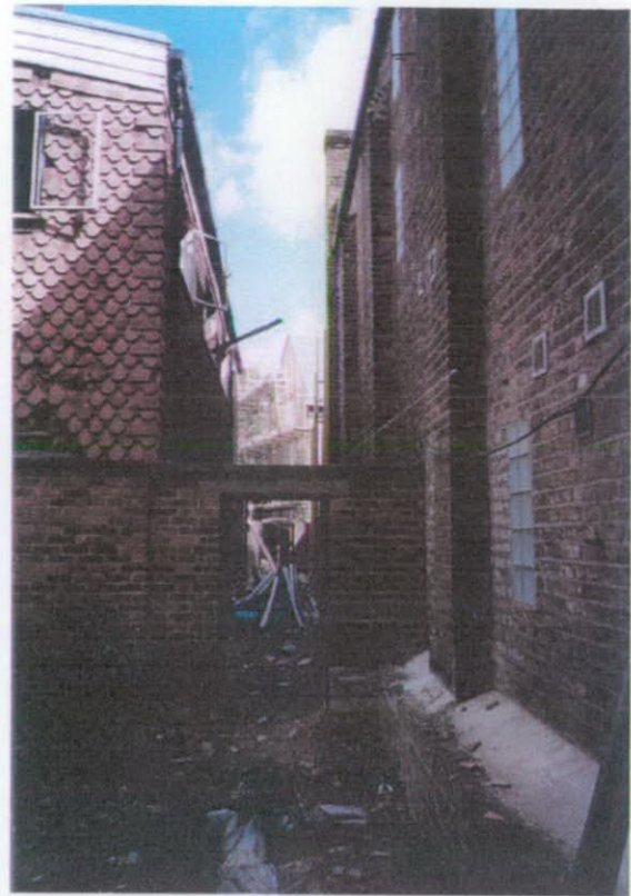
Proximity of the now demolished Sheepshank Public House to the organ factory
