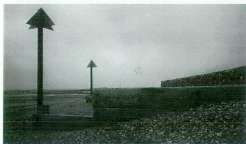
Gabion and timber 'groynes'
