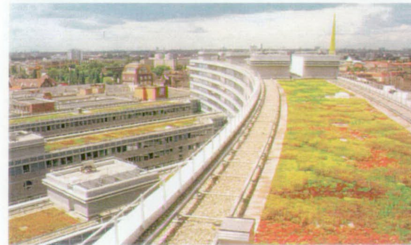
Extensive Roof Garden
