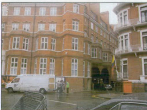
Knightsbridge Crown Court - Service Access
