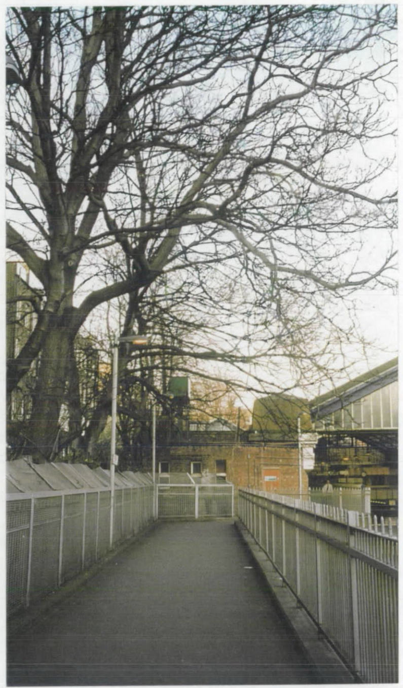
High Level Walkway Uncovered Section
