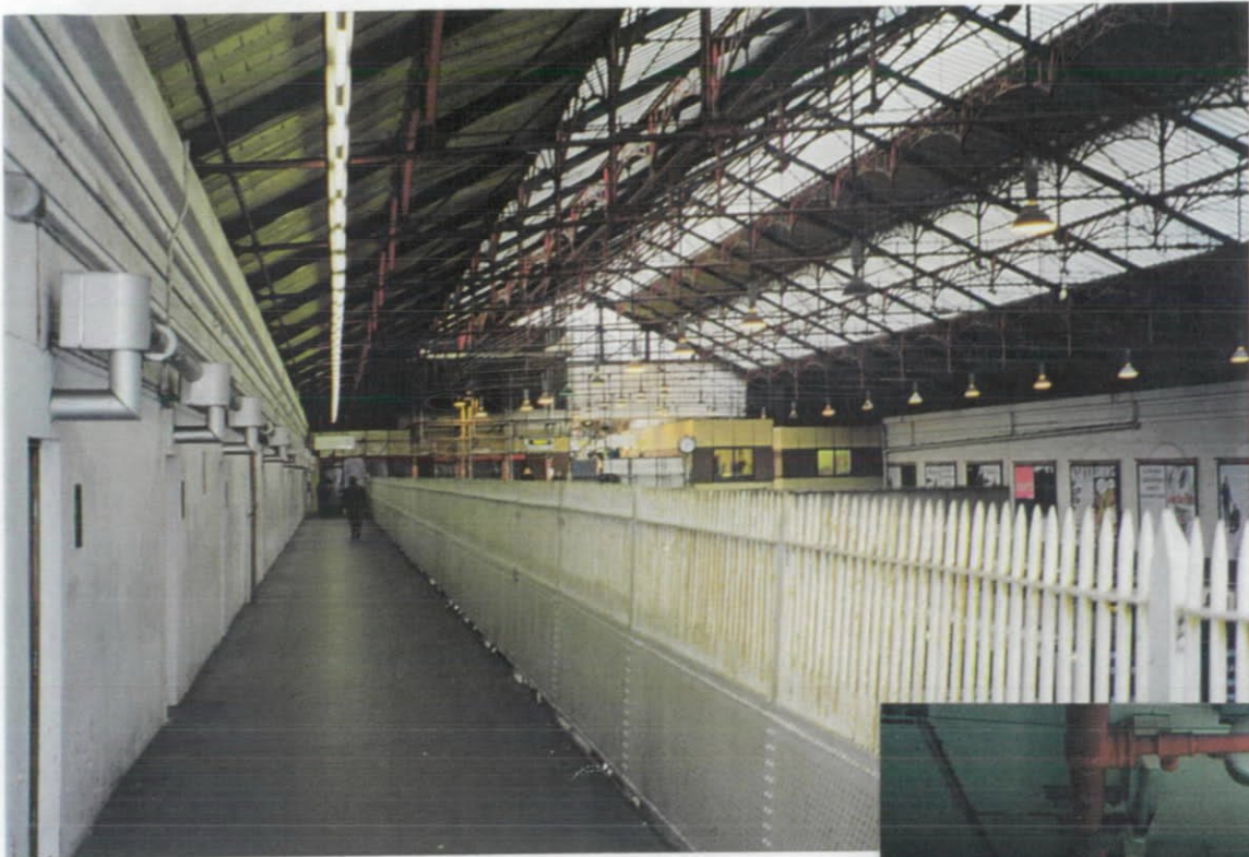
High Level Walkway Covered Section
