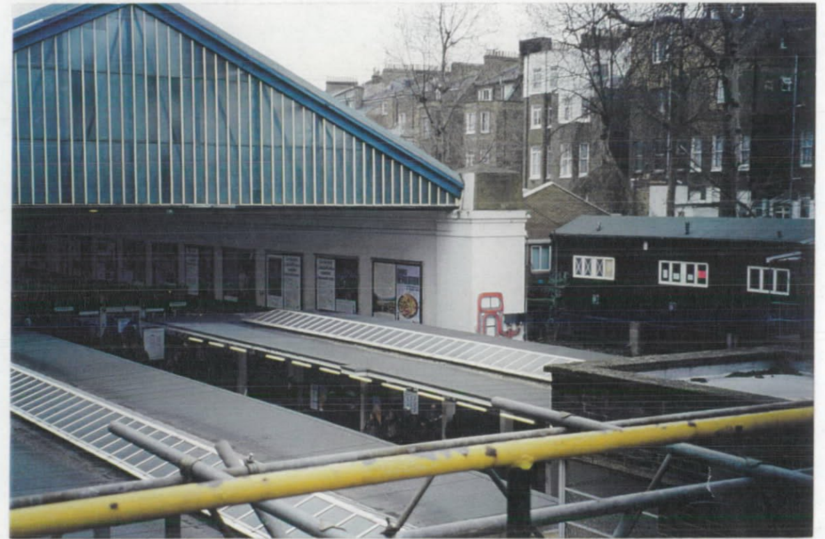
District Line Canopies
