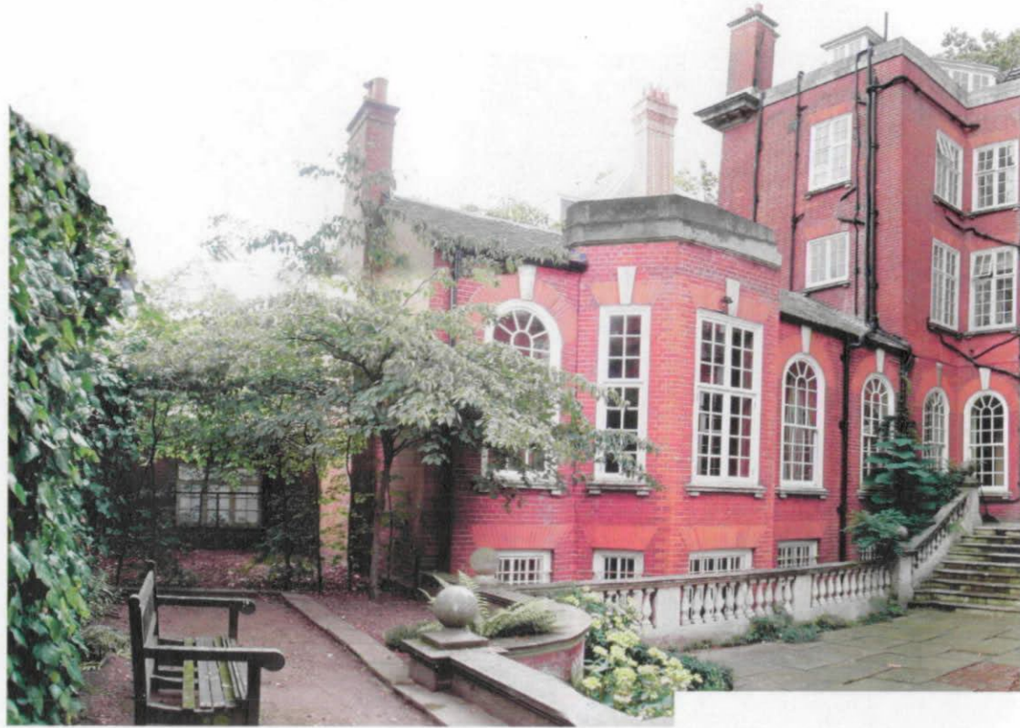
01 existing view of rear garden
