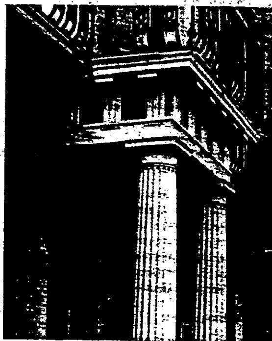
Restored porch in Royal Crescent, W11.
