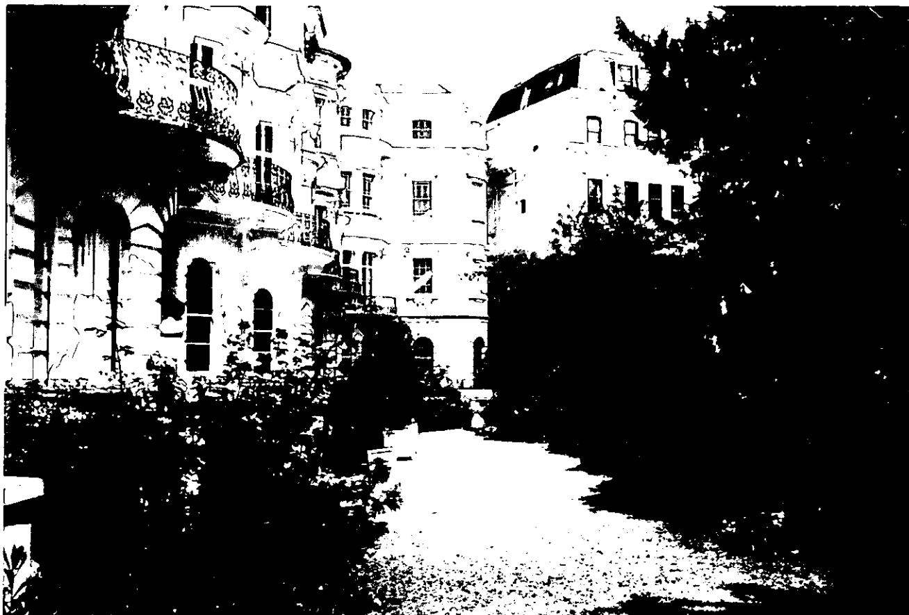
Detailed design of rear elevations of some terraces has resulted in a façade of equal importance to the front.
