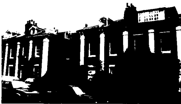
An alteration replacing an attractive dormer window and disrupting the symmetry of the pair of houses.
