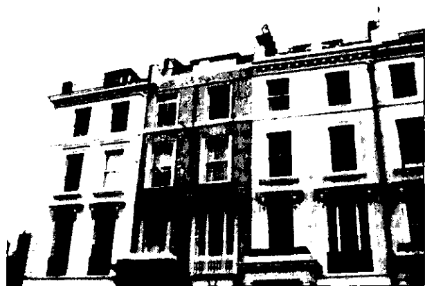
Loss of crowning balustrade, obtrusive wires and alarms detract from the visual quality of the terrace.
