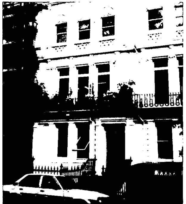
Restoration of original windows would enhance the character of this façade
