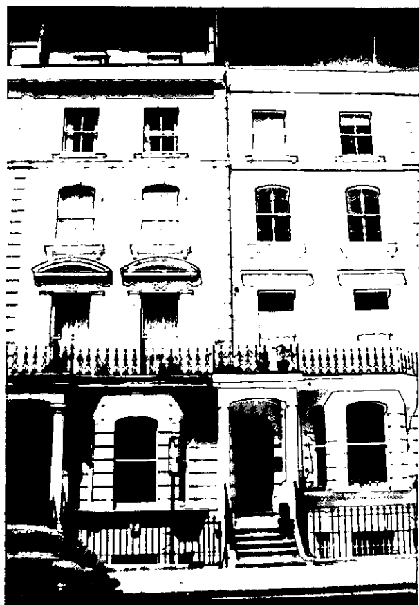
Loss of architectural detail detracts from the house on the right and breaks the continuity of the terrace.
