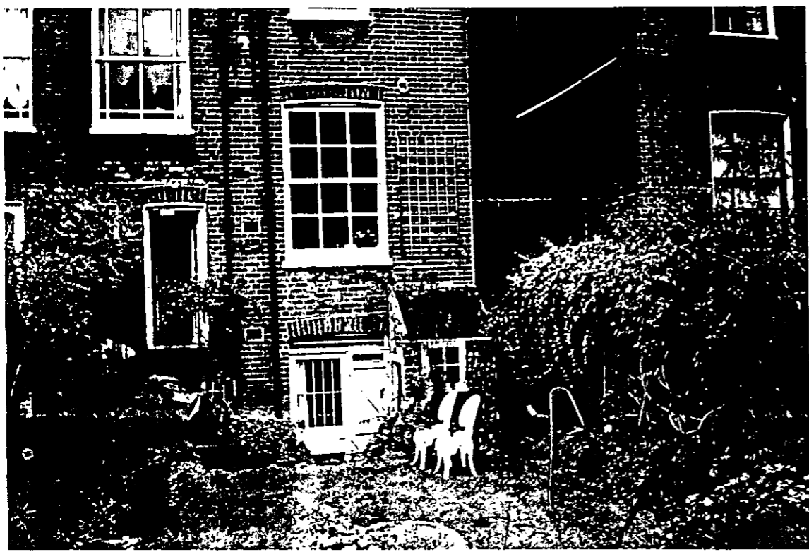
REAR OF NUMBER 24 AT GARDEN LEVEL
