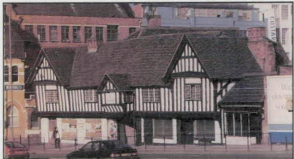
▲ The Old Crown - the oldest pub in Birmingham - faces the Custard Factory Quarter. It is not in a good state of repair.
