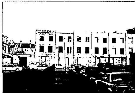
Looking North at previous construction with part of RNIB to the East
