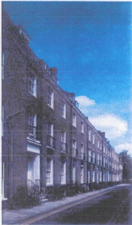
Figure 5 In Georgian streets the small spacing-to-height ratio is compensated for by tall windows. Note how window-head height increases for the lower floors which are more heavily obstructed
