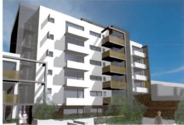
PROPOSED RESIDENTIAL DEVELOPMENT AT 130-136 BARLBY ROAD AND 6 EXMOOR STREET, NORTH KENSINGTON, W10
