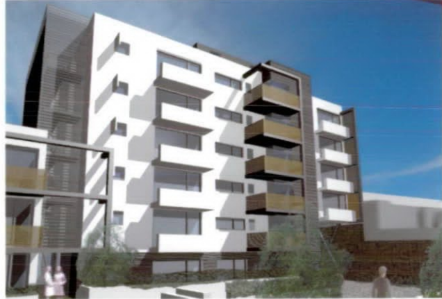
PROPOSED RESIDENTIAL DEVELOPMENT AT 130-136 BARLBY ROAD AND 6 EXMOOR STREET, NORTH KENSINGTON, W10
