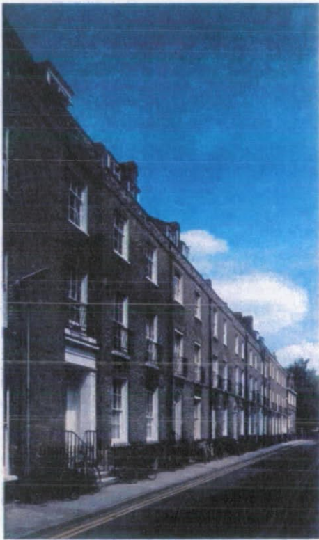
Figure 5 In Georgian streets the small spacing-to-height ratio is compensated for by tall windows. Note how window-head height increases for the lower floors which are more heavily obstructed
