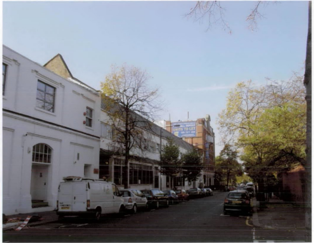
FIG 3. EXISTING OFFICES AND WAREHOUSE AT 130 -136 BARLBY ROAD BUILDING
