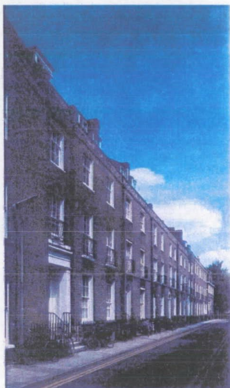
Figure 5 In Georgian streets the small spacing-to-height ratio is compensated for by tall windows. Note how window-head height increases for the lower floors which are more heavily obstructed
