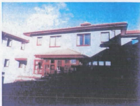
Figure 17 Extensive shadowing can occur in courtyards unless care is taken in their design
