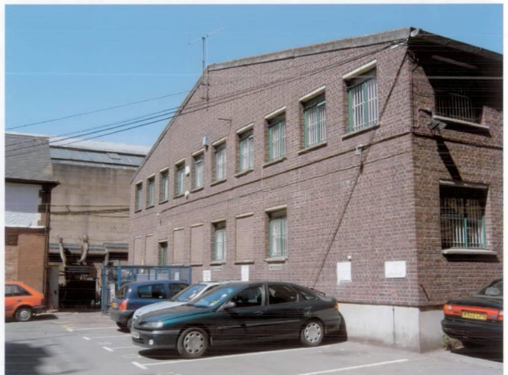
FIG 4. EXISTING TV STUDIOS, 6 EXMOOR STREET
