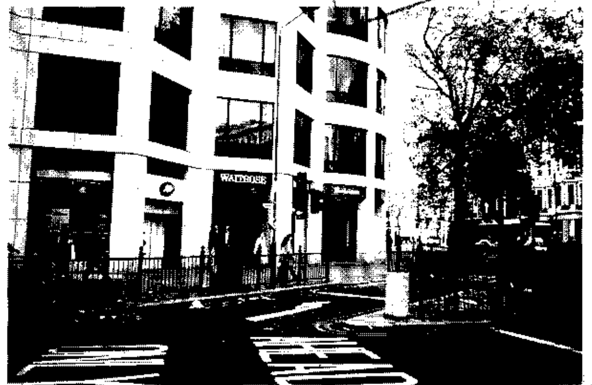
ENTRANCE AT NORTH END OF MALL GENERAL VIEW ACROSS GLOUCESTER ROAD
