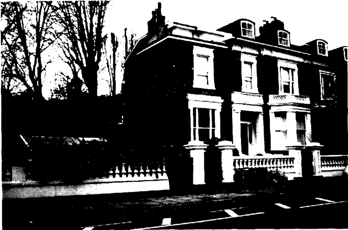
CORNER VIEW - 14 ADDISON CRESCENT
