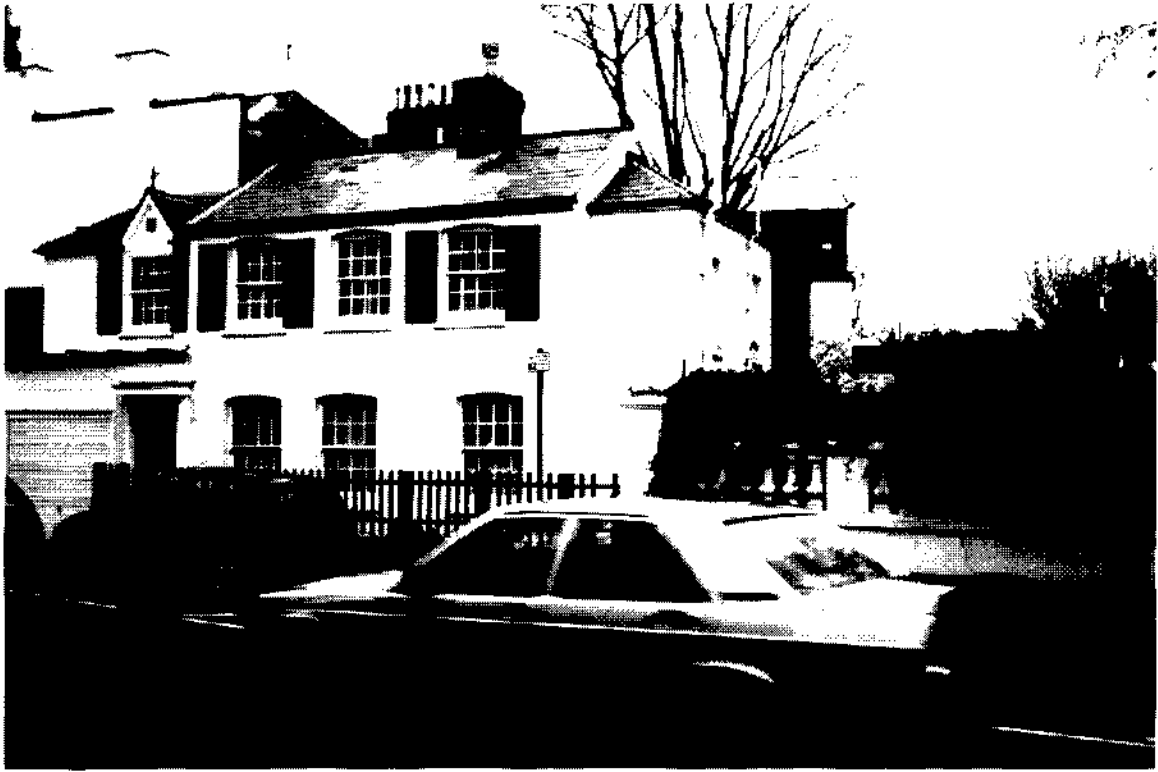
CORNER VIEW - 14A ADDISON CRESCENT - WEST END
