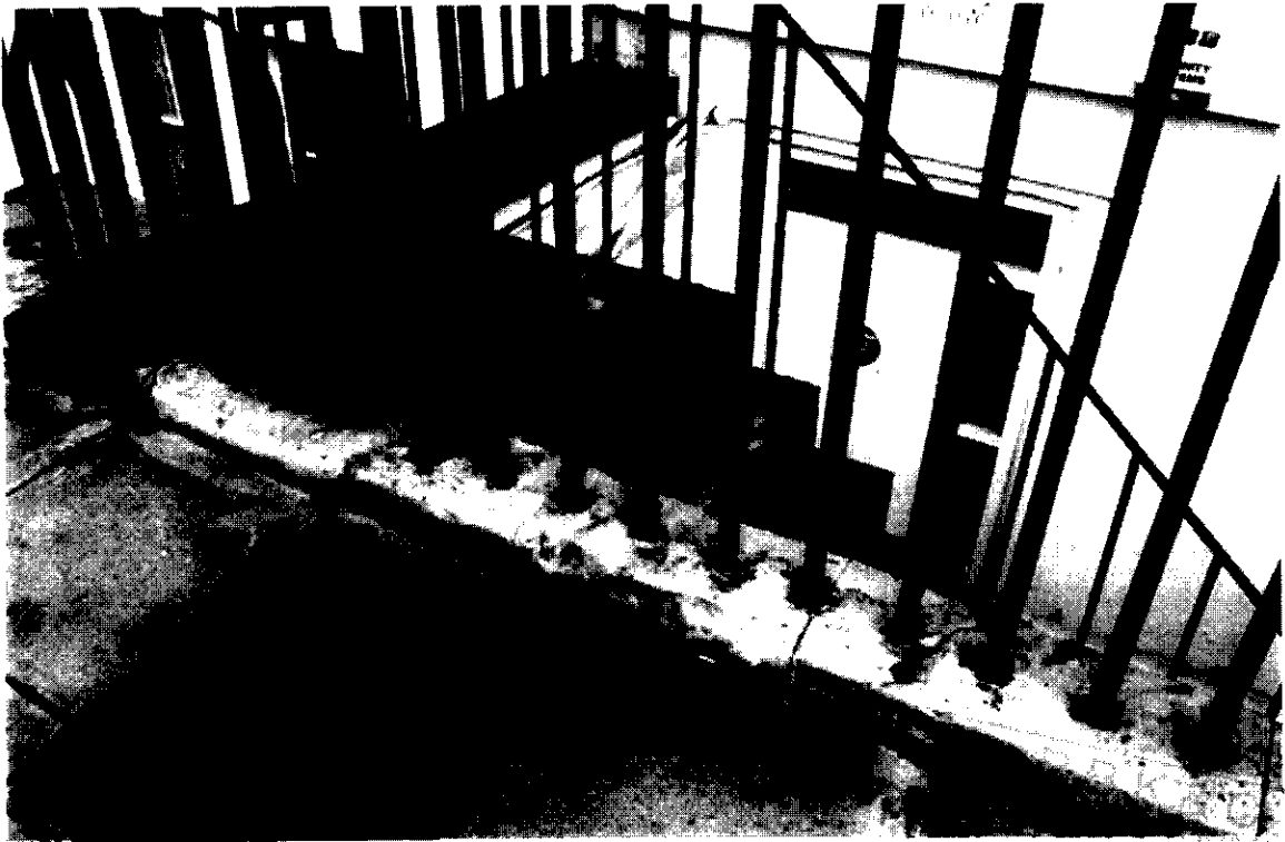
19. First/Second Floor ½ Landing
