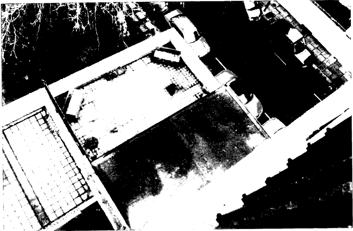
6. Rear terrace. Quarry tiles to be replaced with Yorkstone slabs
