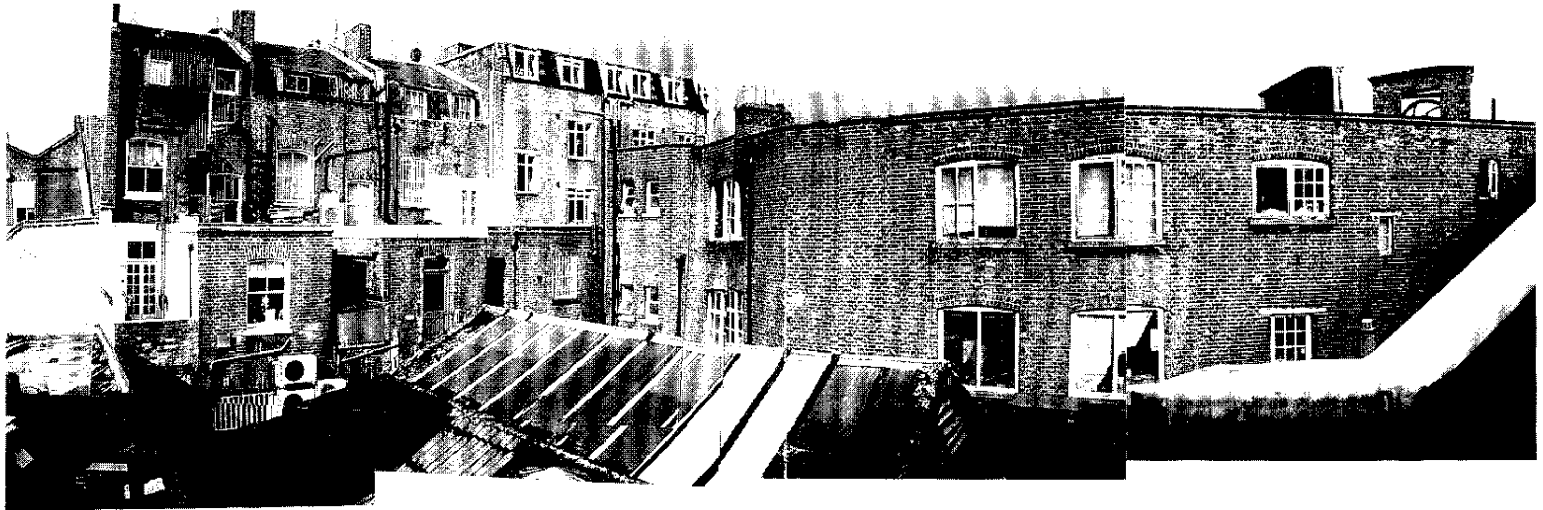
VIEW LOOKING NORTH WEST SHOWING EXISTING GARAGE ROOF AT THE REAR OF THE SITE
