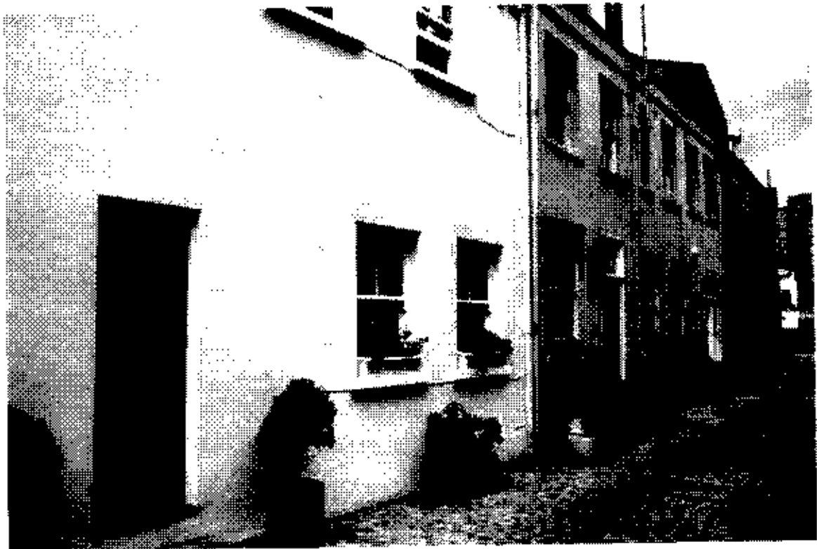
NO 14 LOOKING TOWARDS NO 13
