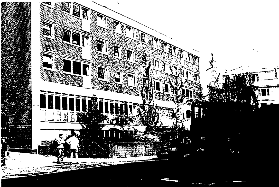
Figure 9b WATER TOWER HOUSE (Campden Hill Road) & 25 CAMPDEN HILL GARDENS, corner of Aubrey Walk/ Campden Hill Road.
