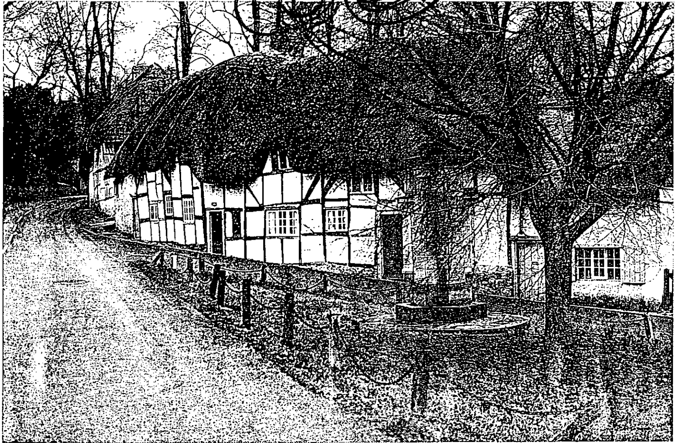
Wherwell, Hants Vernacular building traditions like timber frame construction or thatching techniques should be studied and recorded. (Geoff Noble)
