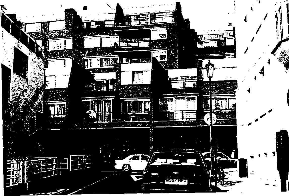
Figure 10a. KENSINGTON HEIGHTS (Campden Hill Road) seen from Peel Street.
