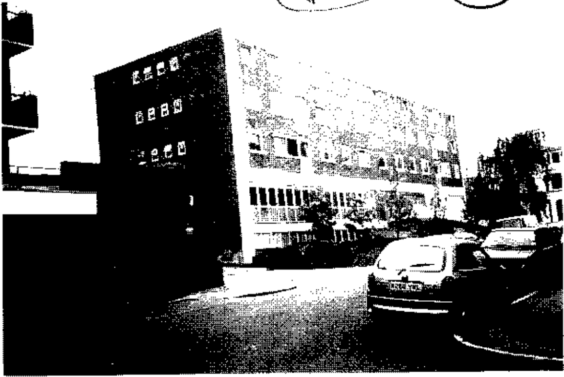
9. RT REF 19/1/9916/9.5.99 Looking north-west at front and side of 5-storey Water Tower House.
