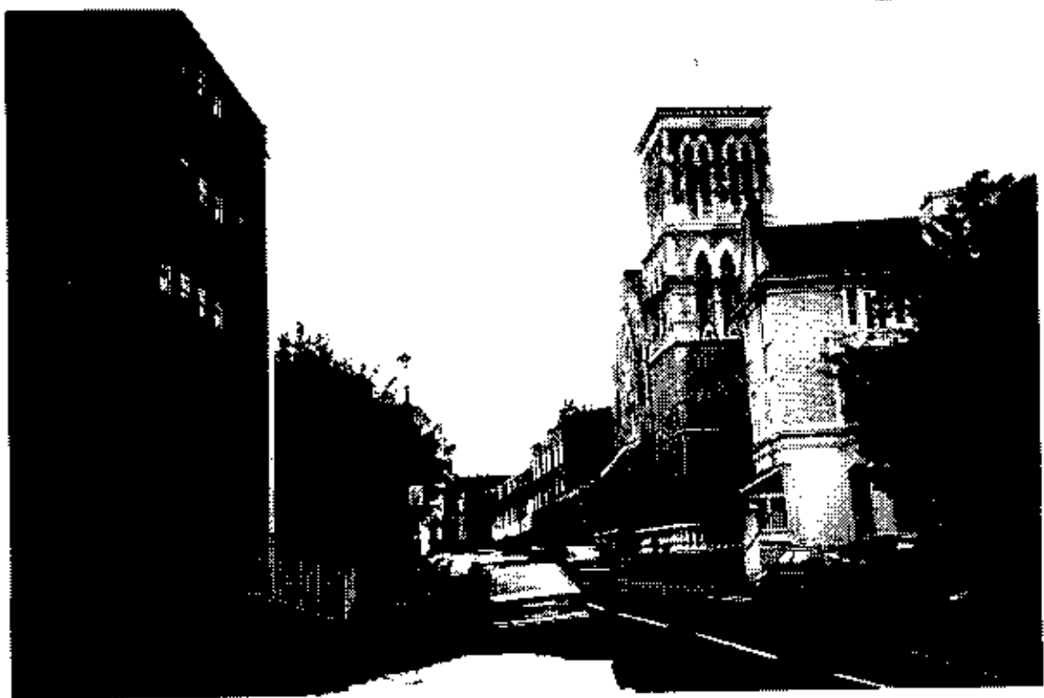
14. RT REF 241.9916/9.5.99 Looking west down Aubrey Walk. 3 listed Georgian houses beyond Bassett Keeling's listed St. George's.
