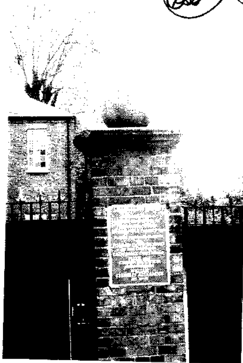
55. RT REF 7/1/9916/9.5.99 Entrance to Aubrey House at western end of Aubrey Walk.
