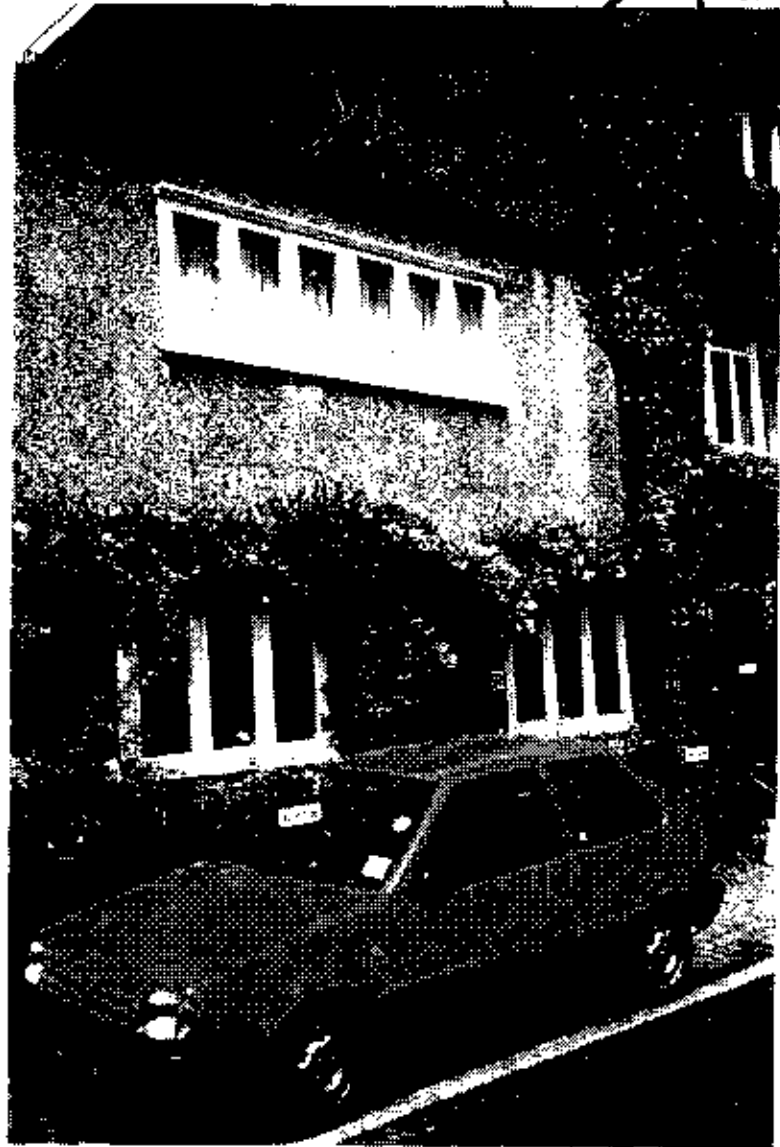
62. RE REF 9/4/99 16:30.5.99 North Side. No. 30. Mews building, now pebble-dashed, with new windows and front door. Parking on cobbled side-walk.
