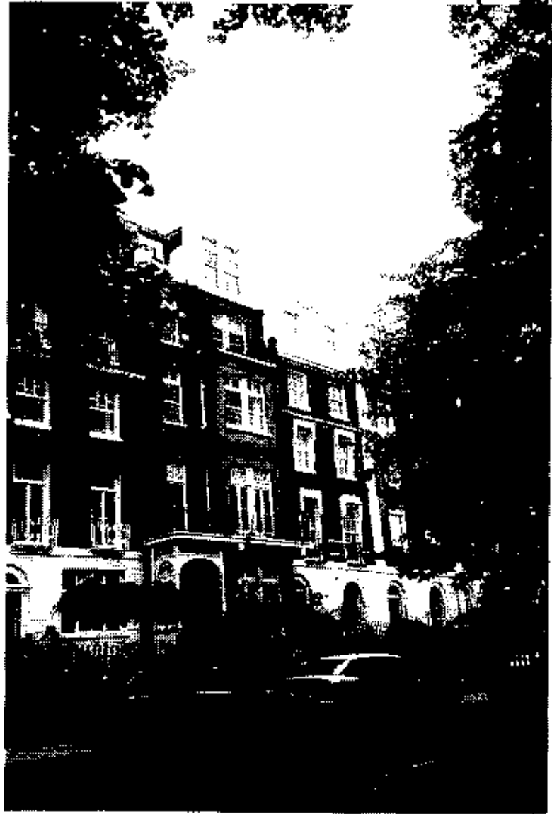
75. RT REF 21/4/9916/30.5.99 South side of Campden Hill Square, mid-Victorian five storey family houses, stock brick with stuccoed ground floors, punctuated here by red brick No. 18, rebuilt by J T Newman in 1887-8.
