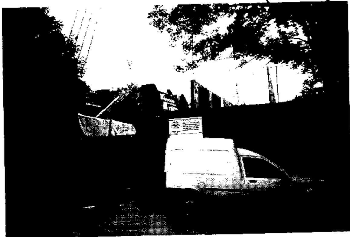
72. RT REF 19/4/9916/30.5.99 South Side. Entrance from Aubrey Walk to Thames Water Site. Appeal Site beyond.
