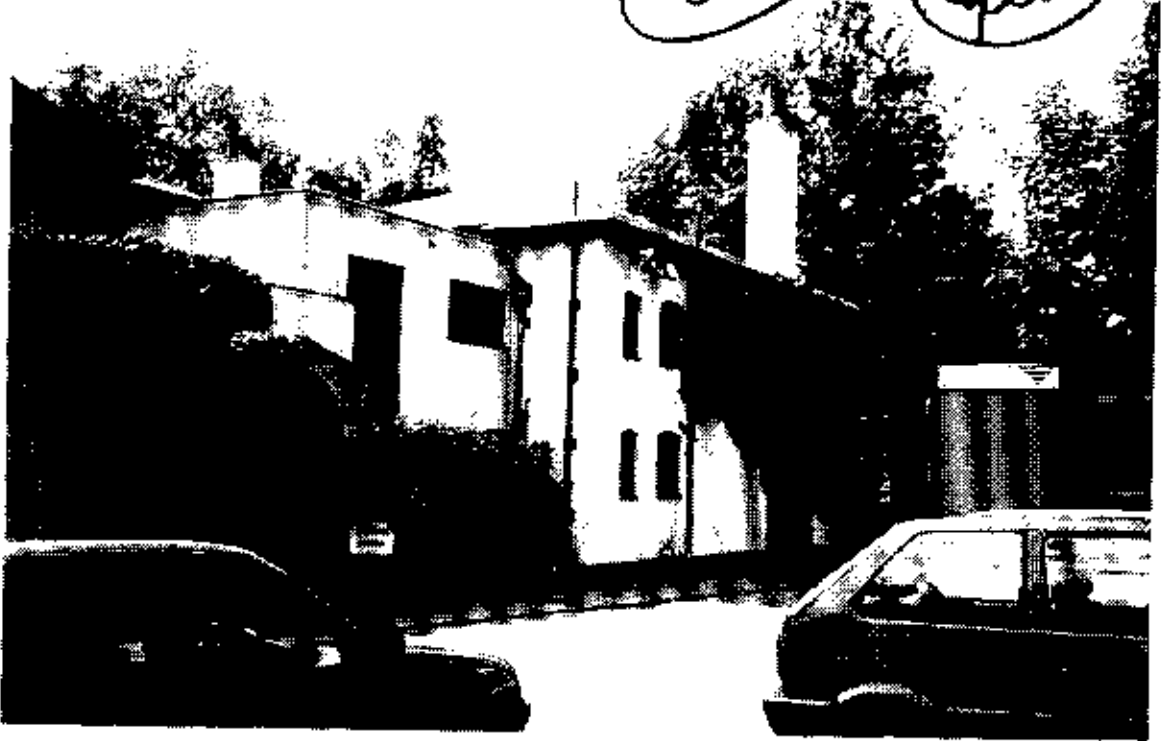
93. RI REF 206/9916/L6.99 North elevation of Thorpe Lodge, from car park. Looking west.
