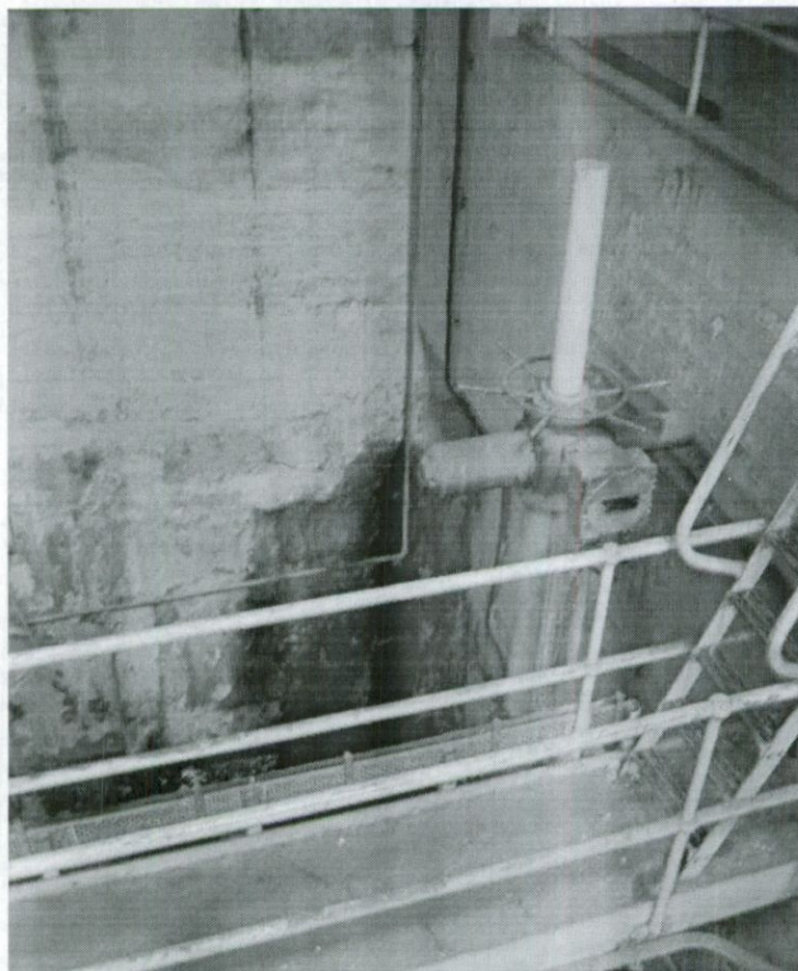
Photograph 6 RBKC Water Ingress within the Deep Trench of the Turbine Hall
