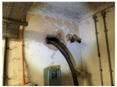
The perimeter walls and doors of the electrical cupboards / risers in the communal lobbies generally appeared to have suitable fire resistance (some riser doors were FD60 and some were FD60S).
