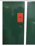
However there was an unsealed redundant lock at the 13th floor with other redundant locks being sealed on the outside of the doors only. To achieve the necessary fire resistance the redundant riser door locks should be sealed on both sides.
