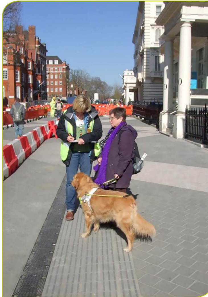
Testing corduroy paving in Exhibition Road
