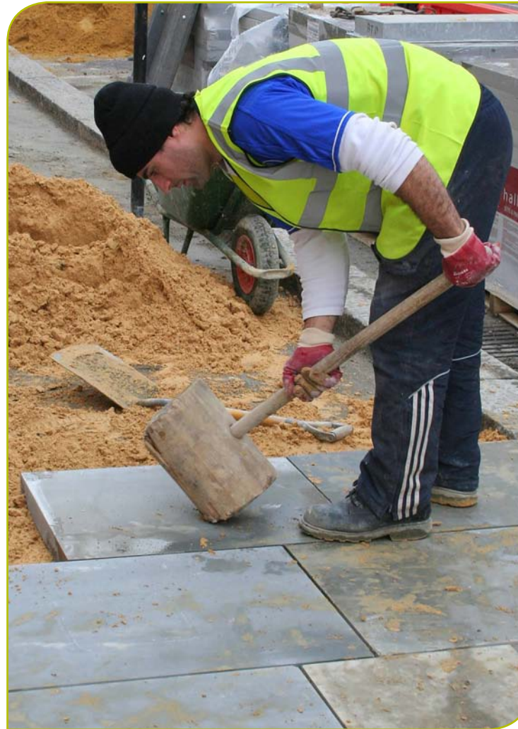
High quality workmanship is essential when laying paving
