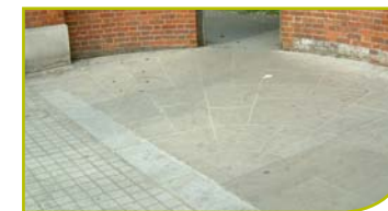
Radial paving detail – Kensington High Street
