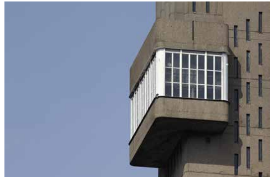
12. Glazing to boiler room external view - RIBA
