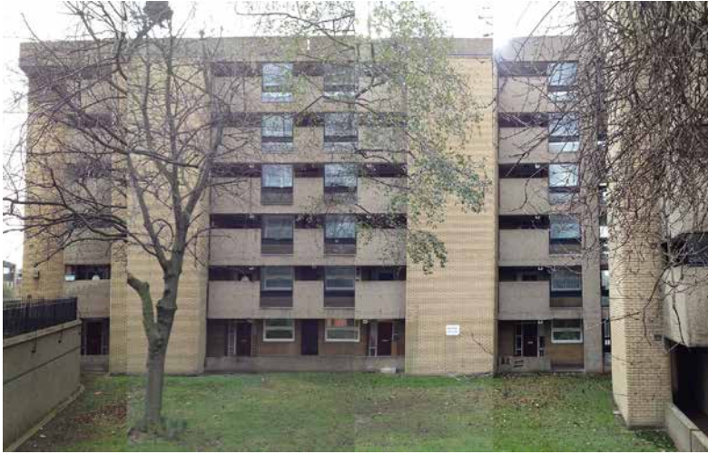
1. Block C, north elevation - HTL 2015
