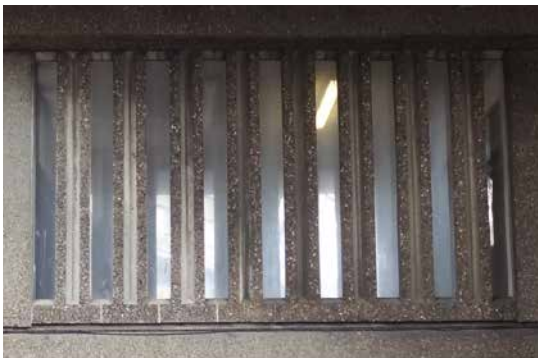
13. Replacement glazing to concrete fins in entrance lobby
