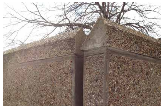
8. Detail of concrete walls - HTL 2015
