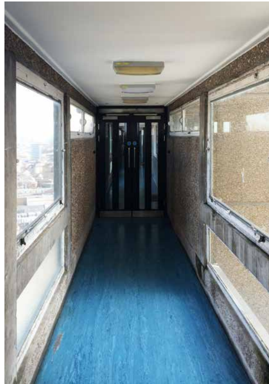
2. Bridge link interior - HTL 2015
