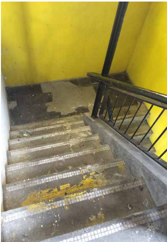
3. Escape stairs current finishes - HTL 2015
