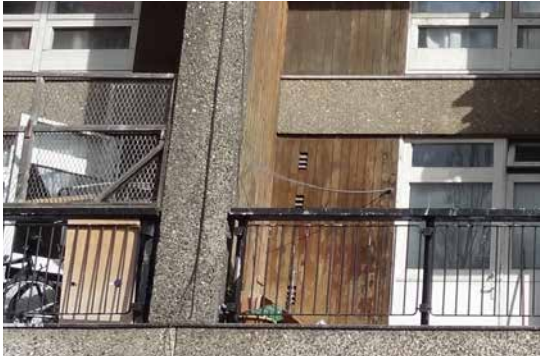
1. Cedar cladding to balconies - HTL 2015
