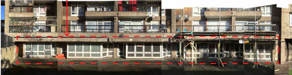
1. South elevation Block A - HTL 2015
