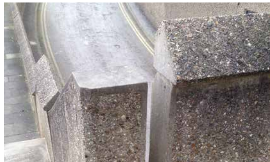
6. In-situ external landscape walls - HTL 2015
