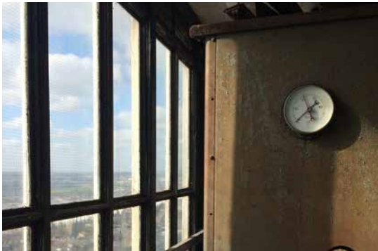
11. Glazing to boiler room internal view - HTL 2015
