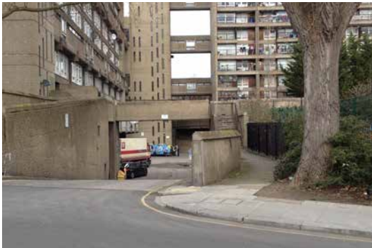
1. Bridge link over service yard - HTL 2015
