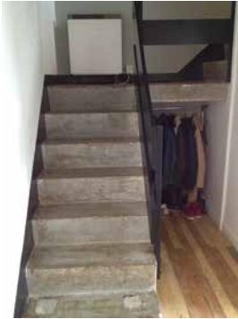
9. Staircase in two bed leasehold flat - HTL 2015
