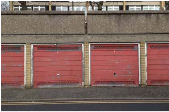
1. Garage elevations - HTL 2015
