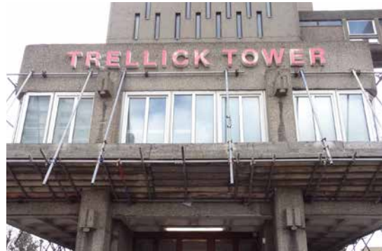
10. Replacement windows to residents' room - HTL 2015
