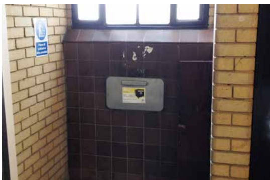
5. Refuse chute - HTL 2015
