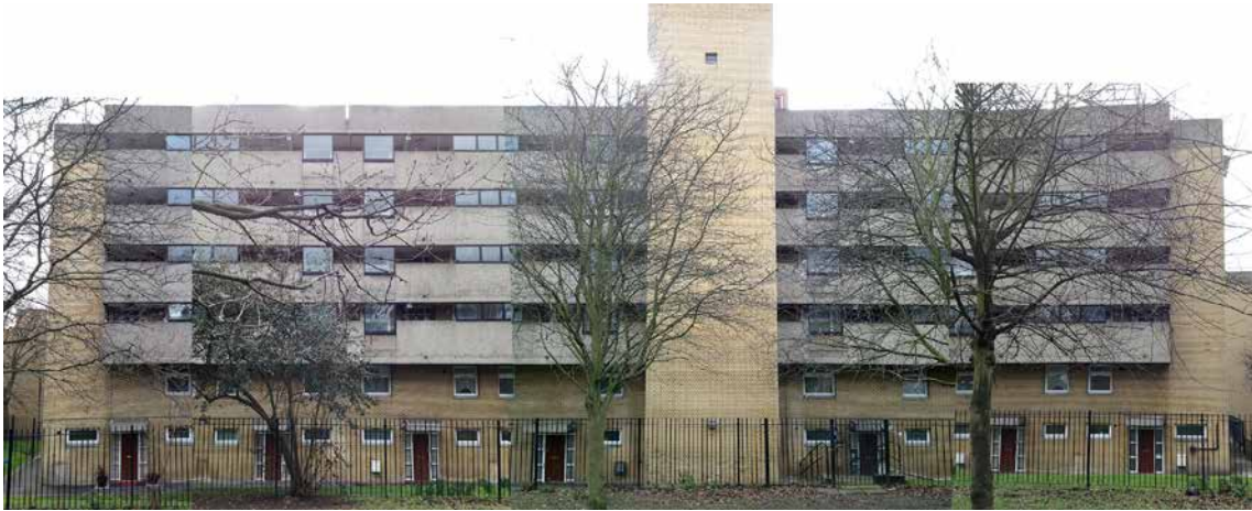
1. Block E north elevation - HTL 2015
