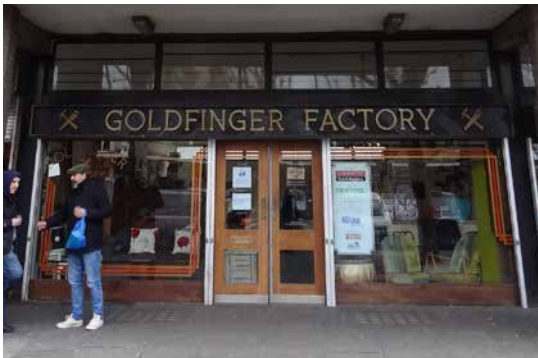
5. Windows to front of commercial units - HTL 2015
