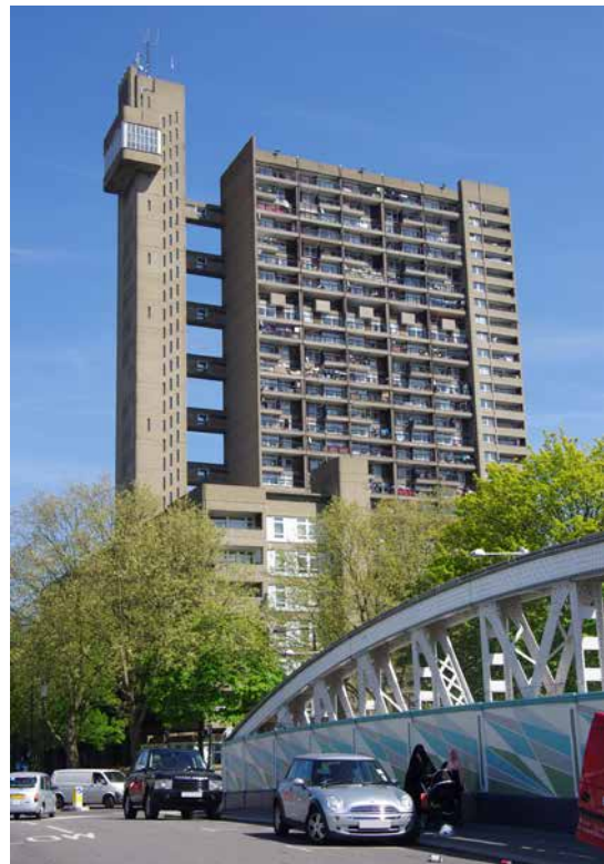
2. Current view from Golborne road bridge - HTL 2015
