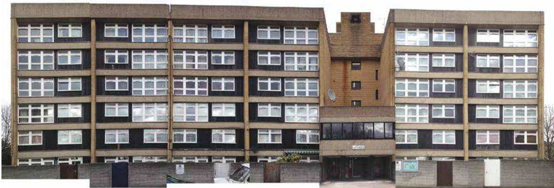
2. Block E south elevation - HTL 2015
