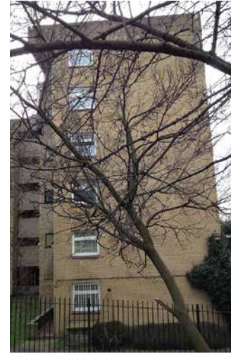
2. Block C, north gable end - HTL 2015
