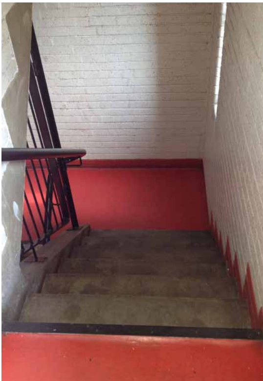
3. New flooring to stair landings - HTL 2015
