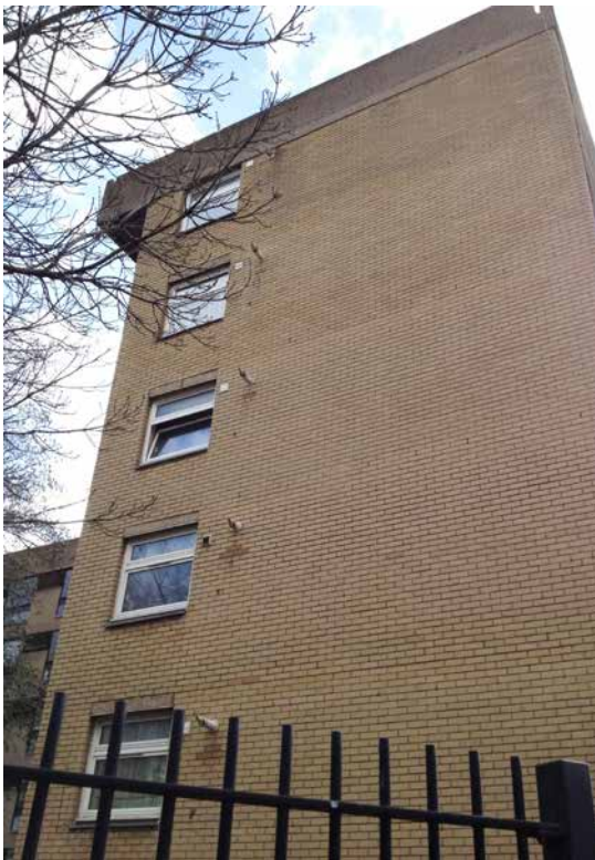
9. Boiler flues to gable end elevation - HTL 2015
