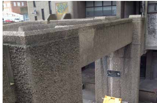
2. Bridge link over service yard - HTL 2015
