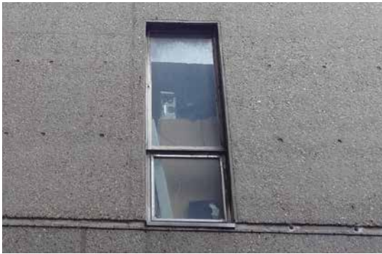
9. Window to Block B north gable end elevation - HTL 2015
