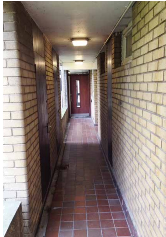
4. Access gallery and flat storage - HTL 2015
