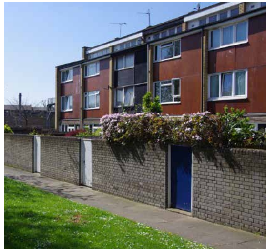
3. Row of rear elevations - HTL 2015
