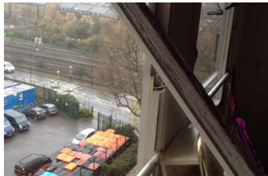
12. Centre pivot opening mechanism - HTL 2015
