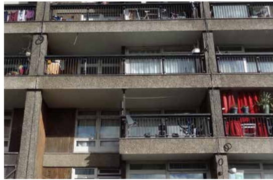
4. Pre-cast panels with exposed aggregate - HTL 2015
