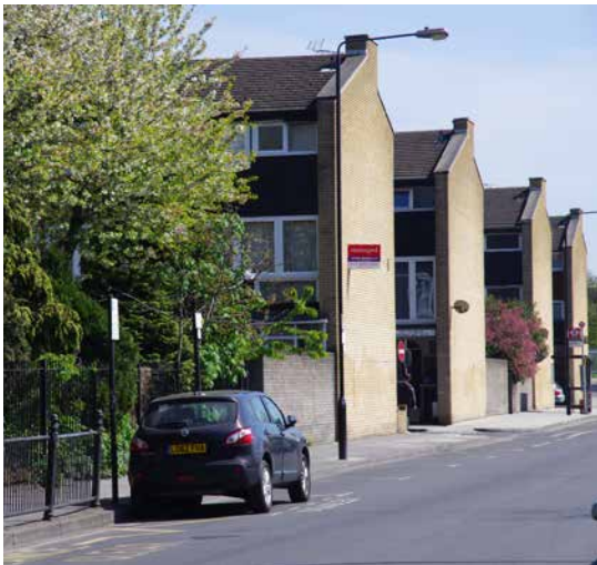
2. Gable end elevations - HTL 2015
