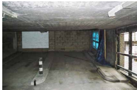
6. Current view inside car parking podium - HTL 2015
