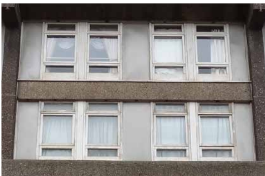
9. Exposed windows on Block A north elevation - HTL 2015
