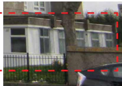
3. West and south elevations Block B - HTL 2015
