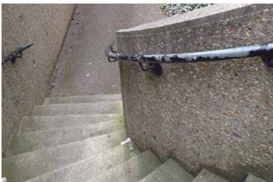
3. Garage stair steps - HTL 2015
