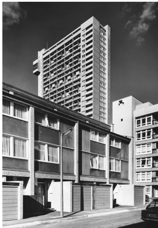
6. View to Trellick with Blocks D and C in foreground - RIBA
