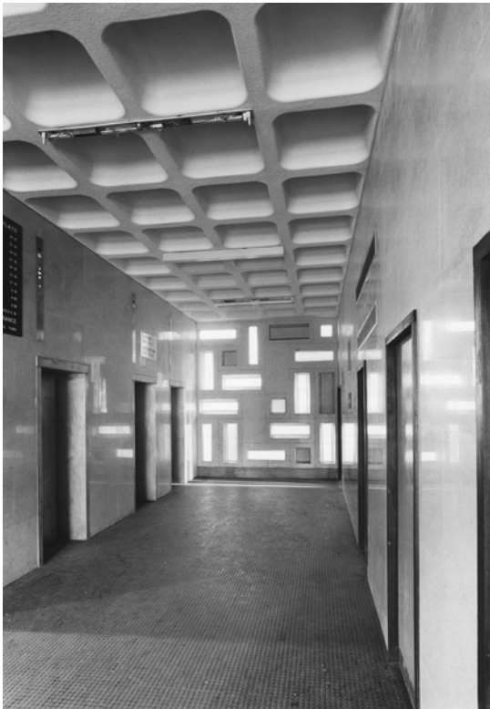
1. Original entrance lobby - RIBA
