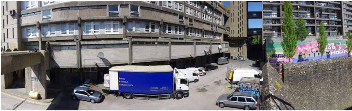
1. Current view of the service yard - HTL 2015
