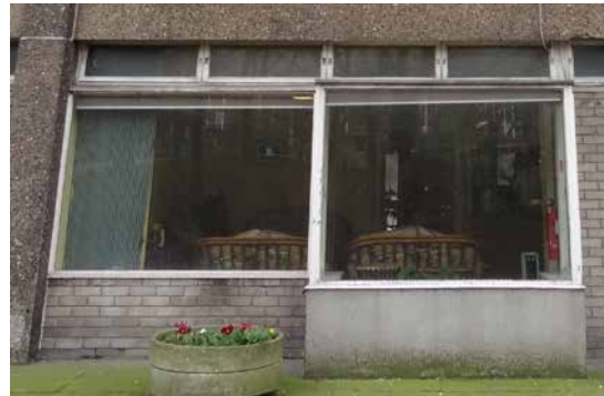
4. Ground floor windows north elevation Block A - HTL 2015
