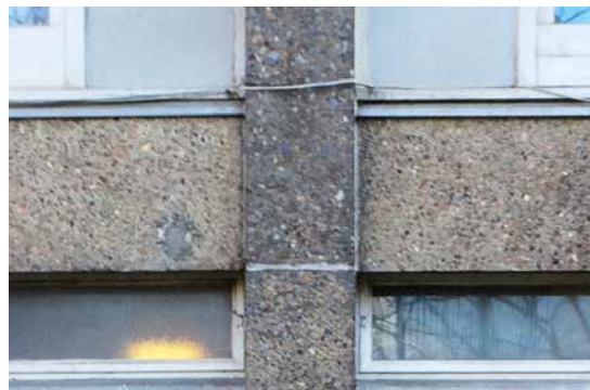
8. Joint to pre-cast panels - HTL 2015
