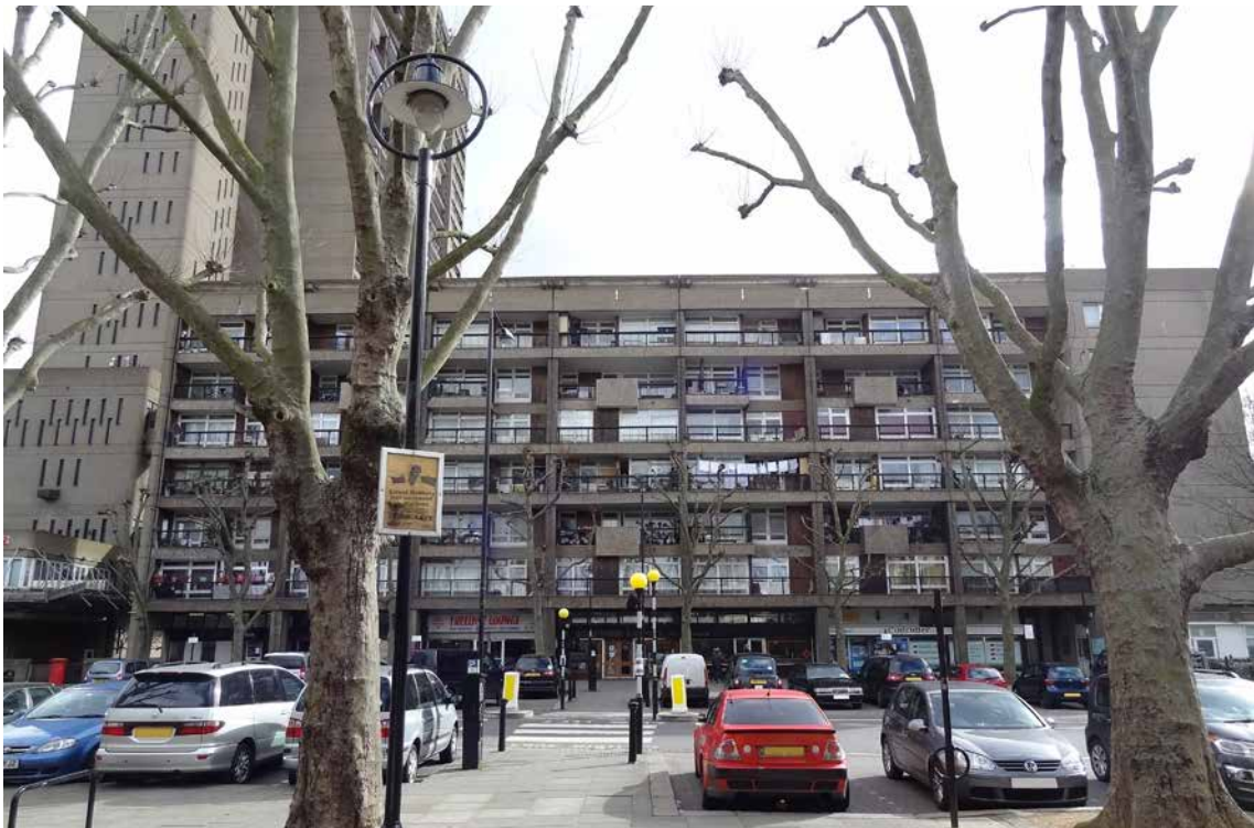
4. The west elevation of Block B from Golborne Road - HTL 2015
