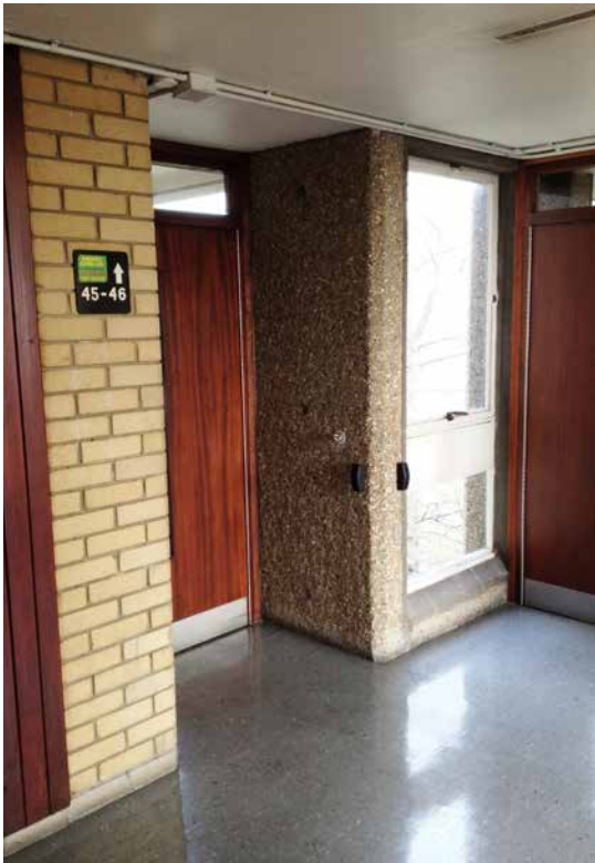
3. Fire door to external access gallery - HTL 2015
