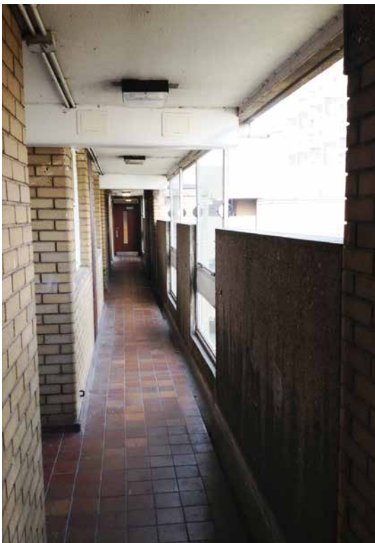
8. Access gallery and boiler flue - HTL 2015
