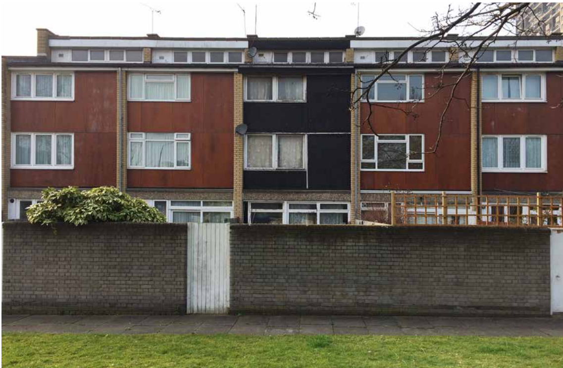
3. Replacement windows and cladding to Block D housing. Note original timber windows and black-stained ply cladding to central dwelling - HTL 2015
