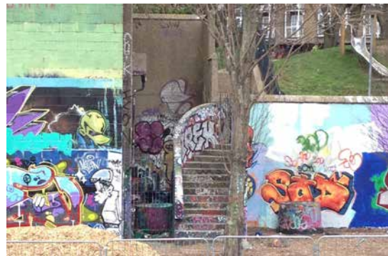
6. Stair to north of courtyard - HTL 2015
