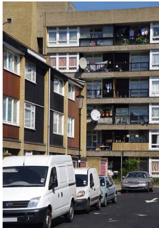
3. View to Block C from Edenham Way terraces - HT 2015
