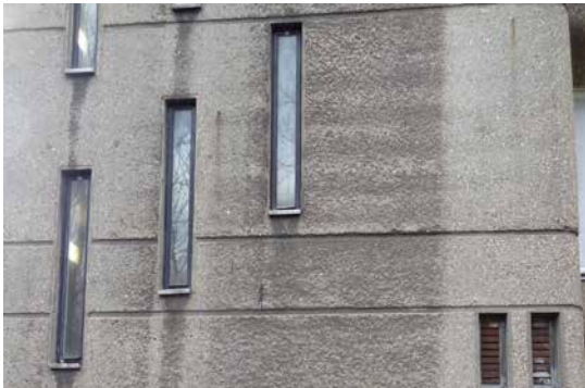
3. Arrow slit windows to service tower - HTL 2015
