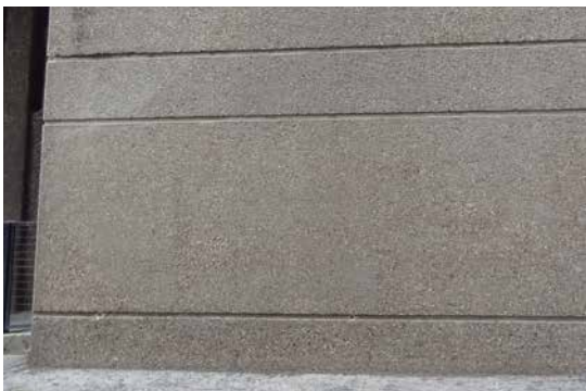
7. Day joint to in-situ concrete - HTL 2015
