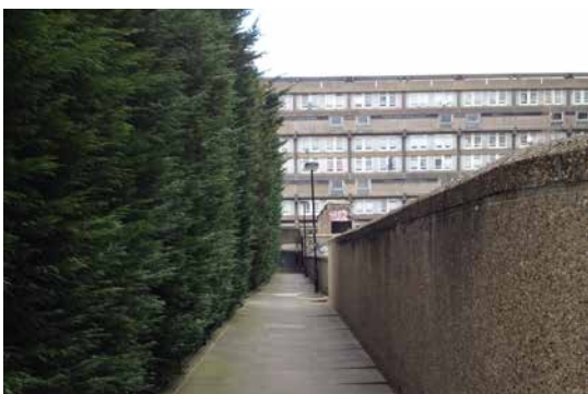
7. Compromised east-west route - HTL 2015
