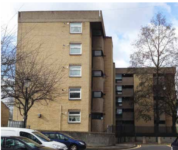
5. Block C, east elevation - HTL 2015
