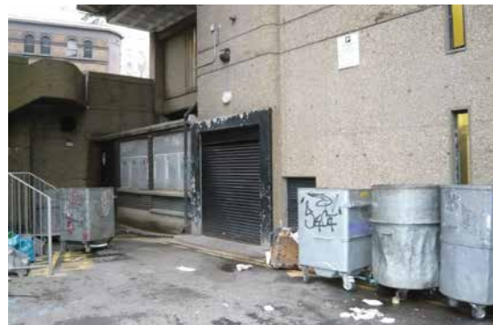
4. Substation and adjacent bin store - HTL 2015
