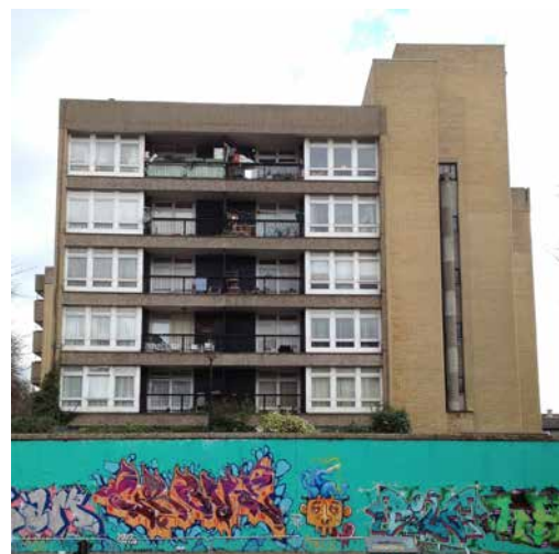
6. Block C, west elevation - HTL 2015
