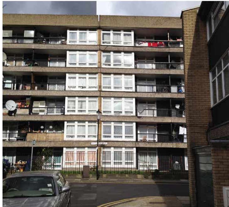
4. Block C, south elevation - HTL 2015
