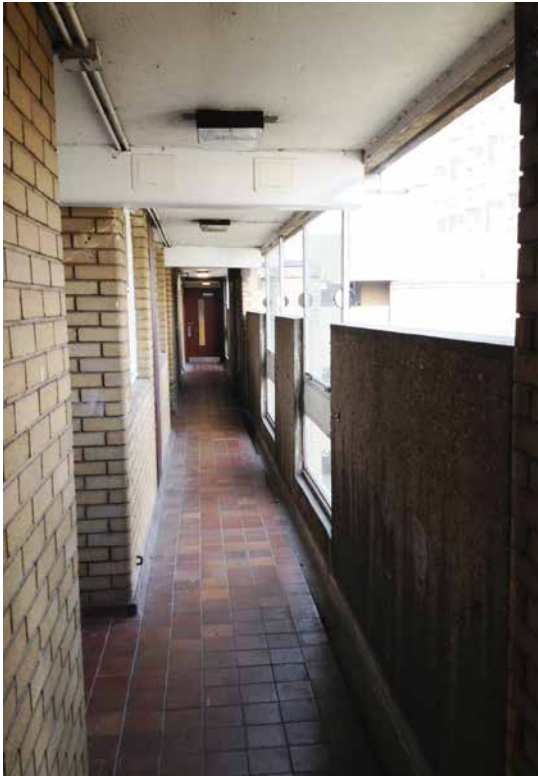
7. Boiler flue on access gallery - HTL 2015
