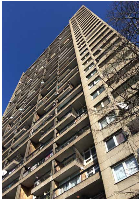
4. South elevation of Block A - HTL 2015
