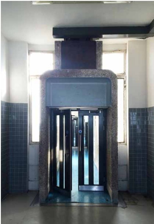
1. Lift lobby fire doors - HTL 2015
