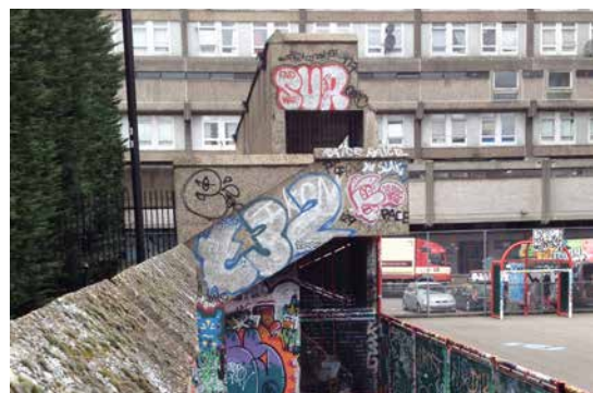
4. Redundant ramped structure - HTL 2015
