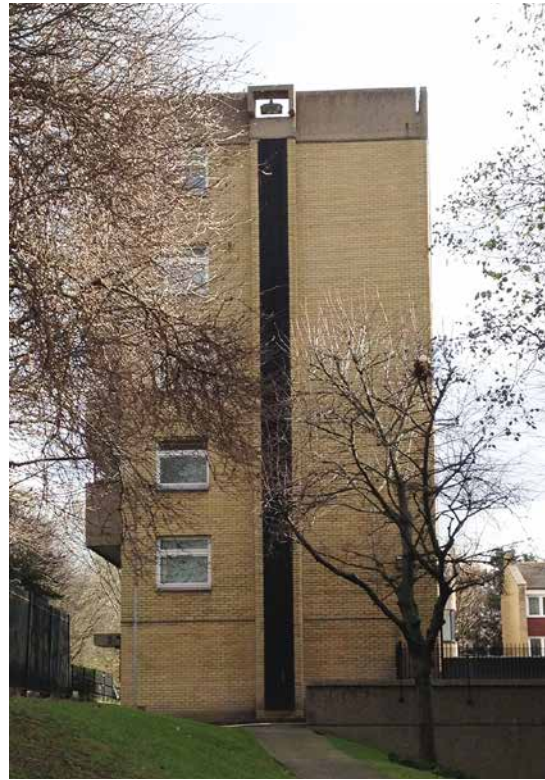
4. Block E west elevation - HTL 2015
