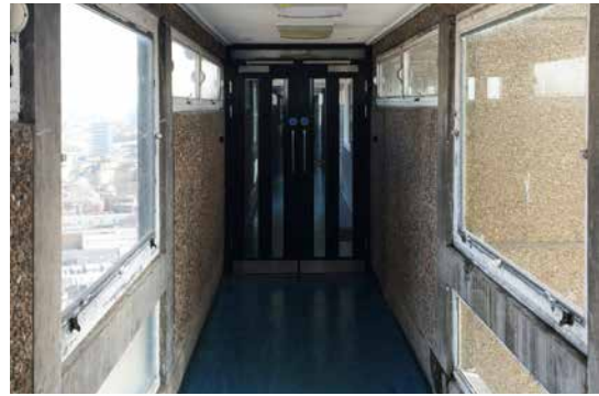
2. Windows to access galleries/ bridge links - HTL 2015
