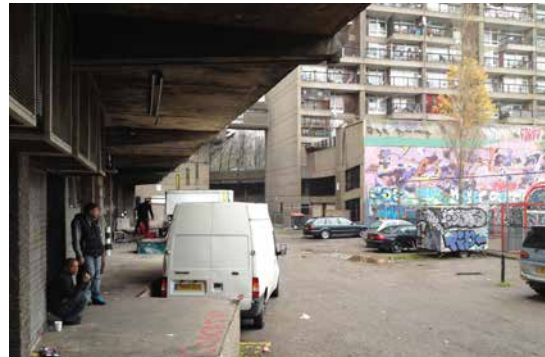
3. View of loading bays - HTL 2015
