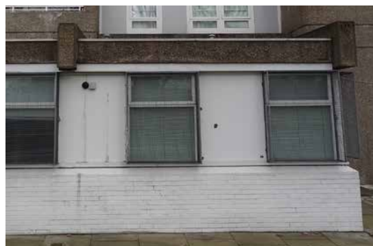
14. Windows to Block B south gable end - HTL 2015
