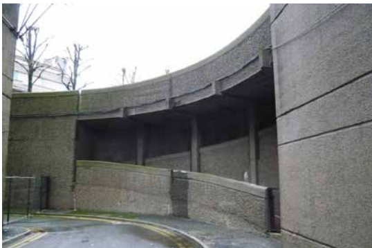
5. Current view of service yard - HTL 2015
