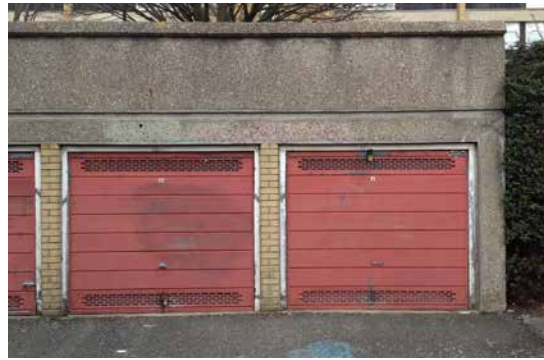
2. Garage elevations - HTL 2015
