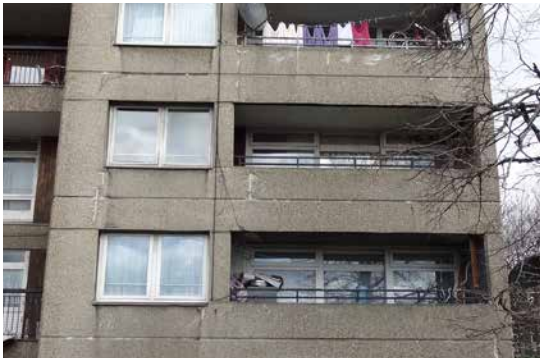
3. In-situ cast external walls with day joint - HTL 2015
