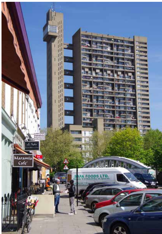
3. Current view from Golborne road - HTL 2015
