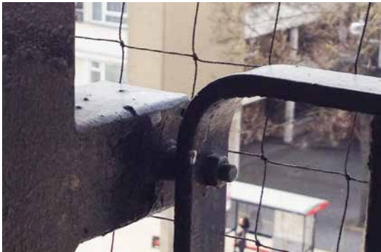
3. Detail of metal railings - HTL 2015
