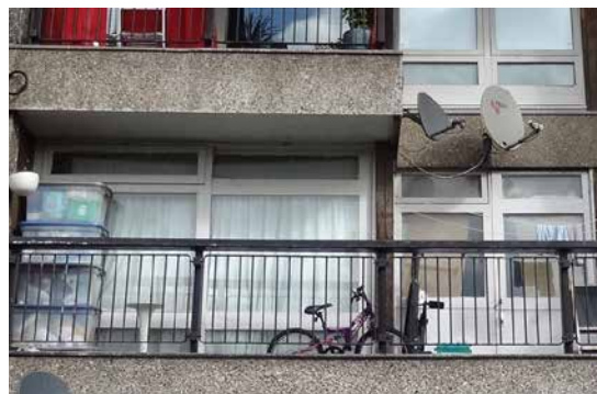
10. Sheltered windows on Block A south elevation - HTL 2015
