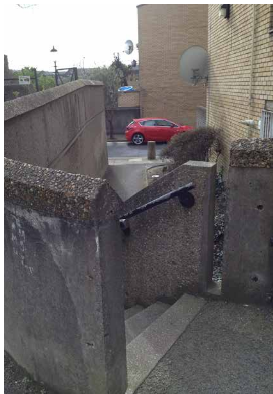
4. Garage stair balustrade - HTL 2015
