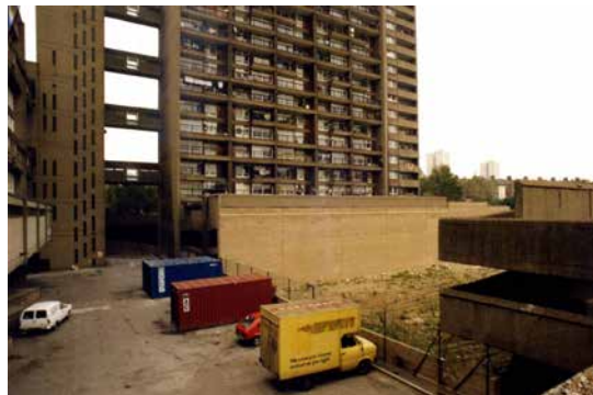
2. The remaining podium after partial demolition - J. Dunnett 1989
