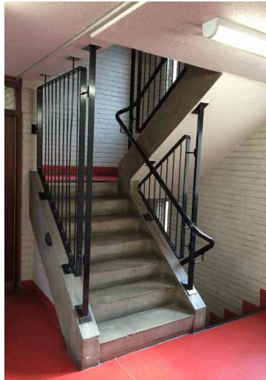
2. Stair and lift lobby - HTL 2015
