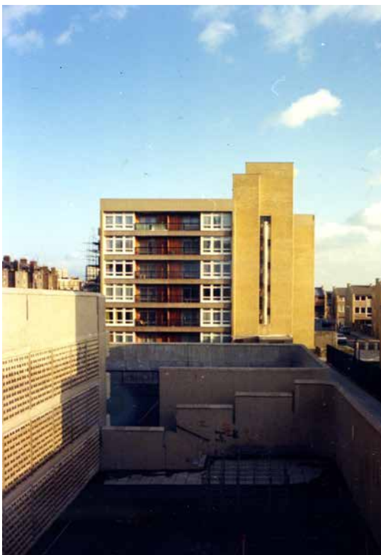
3. Original podium viewed from Block B - James Dunnett
