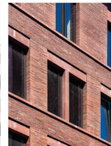
Red brickwork deep reveals and precast lintels and sills
