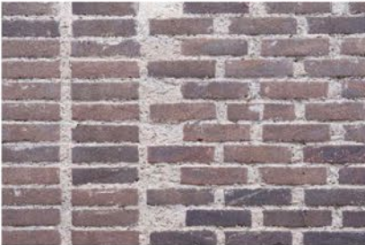
Expressed Mortar Joints & Varying Brickwork
