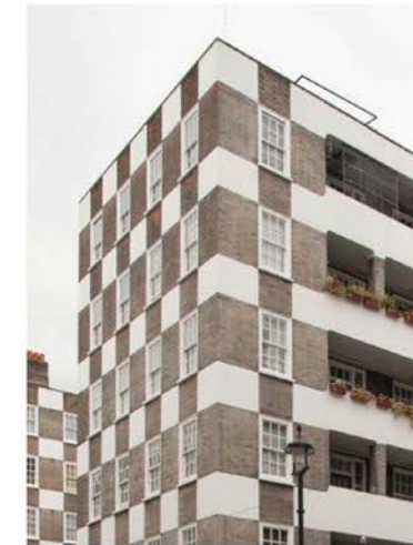
Patterned brick facade and precast solid sided balconies
