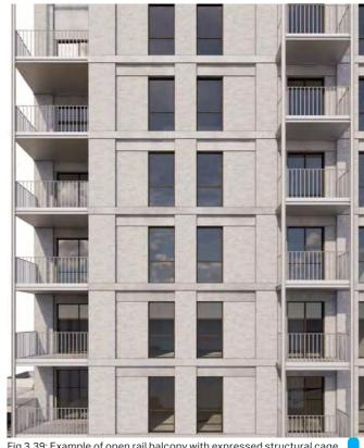
Fig 3.39: Example of open rail balcony with expressed structural cage
