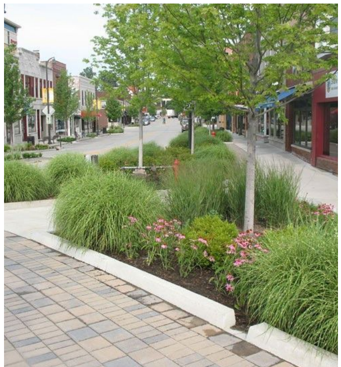
Rain gardens within kerb build-outs
