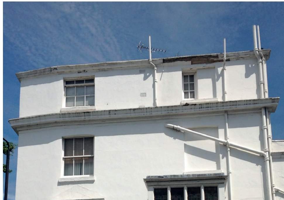
Lack of repairs and maintenance to roof
