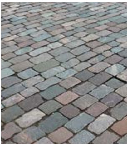
P8 Reclaimed granite setts or similar to RBKC Highways standards
