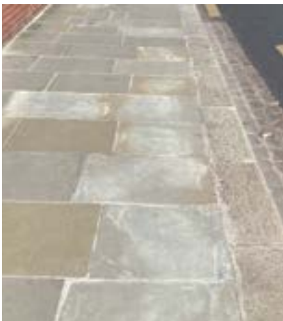
P7 Yorkstone or similar paving and granite kerb to RBKC Highways standards for pavements
