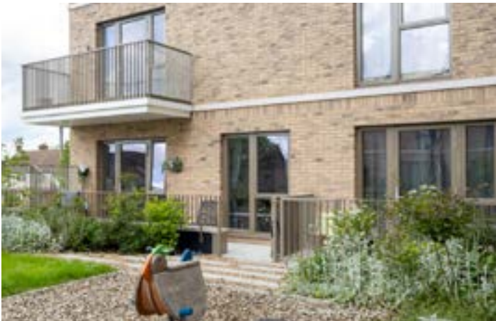
R4, G2/G3 Low metal railing and gate to podium private terraces & podium edge (colour tbc)
