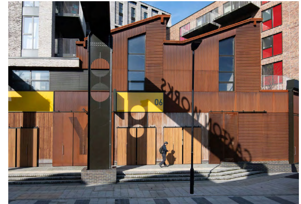
↑ Figure 3.8: Caxton Works, Canning Town: The architectural language is led by the industrial nature of the existing context, and a visually strong ground and first floor keeps the focus on the employment uses at low level. Project by Studio Egret West
