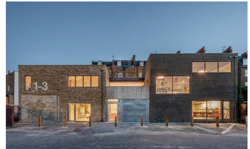
↓ Figure 3.17: Yorkton Workshops, Hackney: the use of a variety of bricks and brick patterns roof form and fenestration distinguish these workshops from the surrounding Victorian residential context. Photo by Taran Wilkhu
