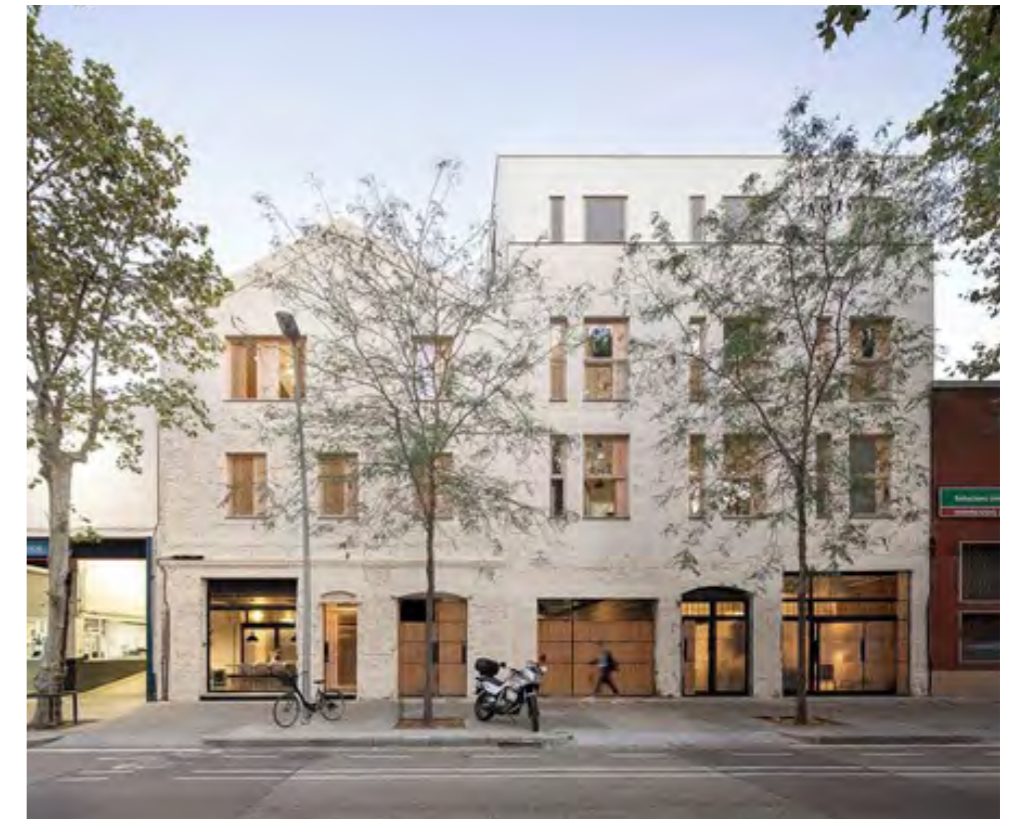
↓ Figure 3.13: Zamness co-working space, Poblenou Cultural and Creative District, Barcelona: varied roof form, set-back upper floor, active frontage and courtyard access. Photo by Del Rio Bani, Zamness Spaces
