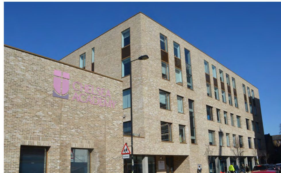
↓ Figure 3.16: Chelsea Academy: High quality and well detailed design using pale soft edged bricks that result in a building that fits sensitively into the existing townscape without copying it
