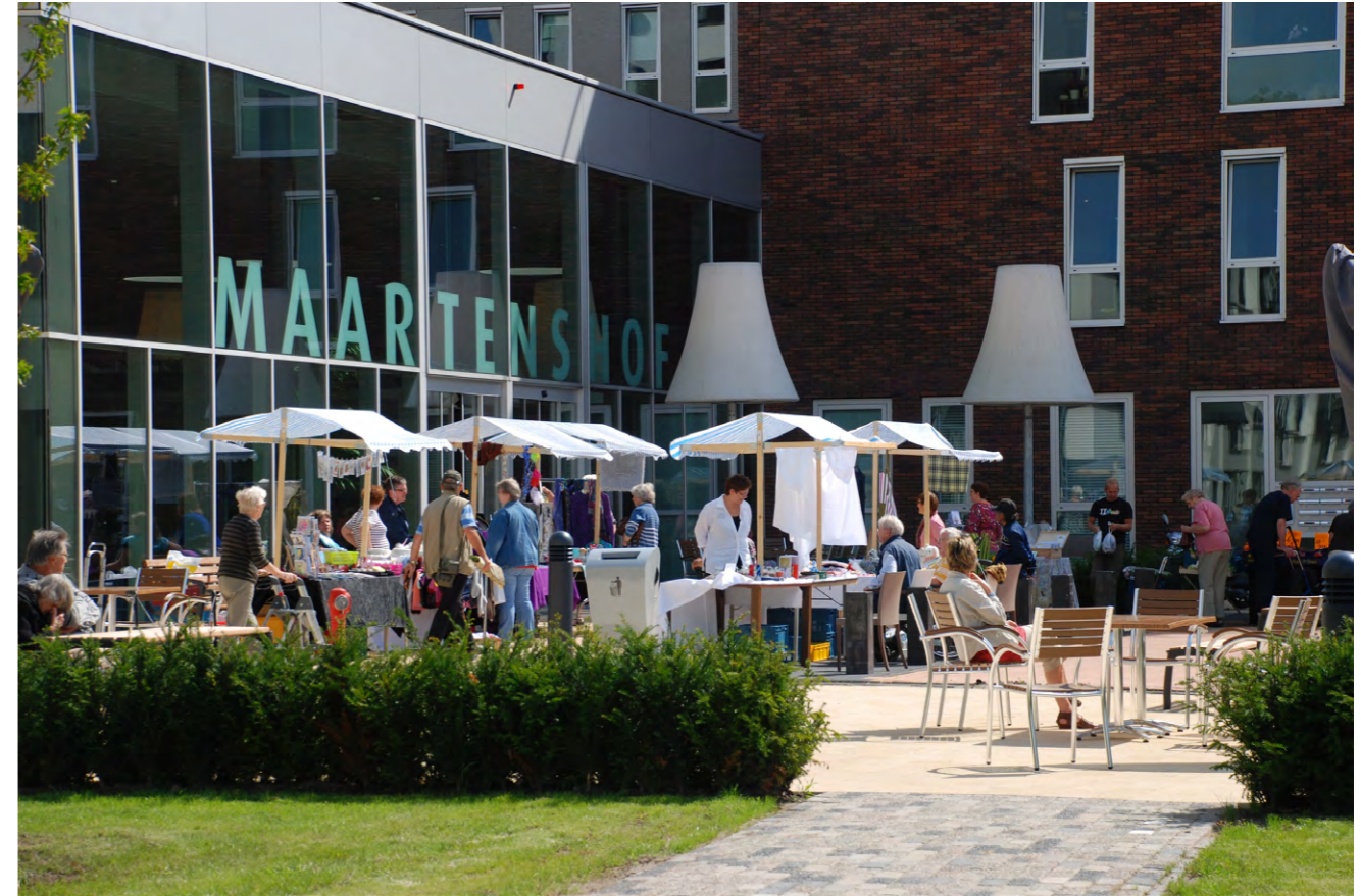
↑ Figure 3.49: Maartenshof continuing care facility's neighbourhood hub in De Rokade Groningen, Netherlands is used by the wider community. Photo © Natalie Willer
