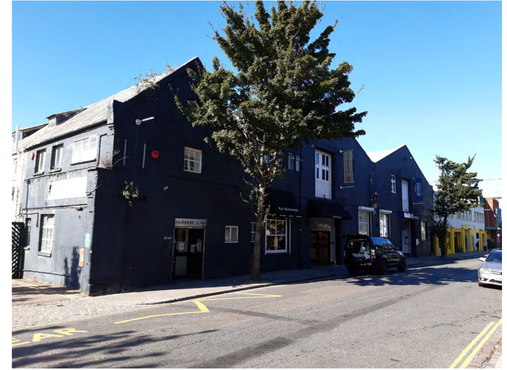
↑ Figure 3.15: Existing buildings on site with characterising 'M' shaped factory roofs and painted brick.
