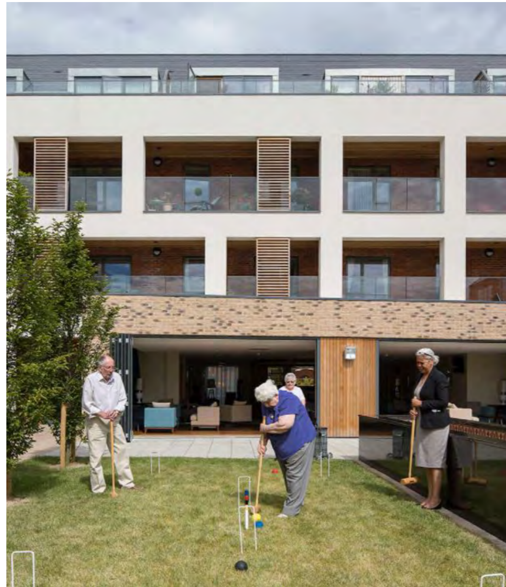
↓ Figure 3.48: Private balconies, communal gardens and connecting indoor communal space at St Bede's Extra Care in Bedford. Project by PRP Architects
