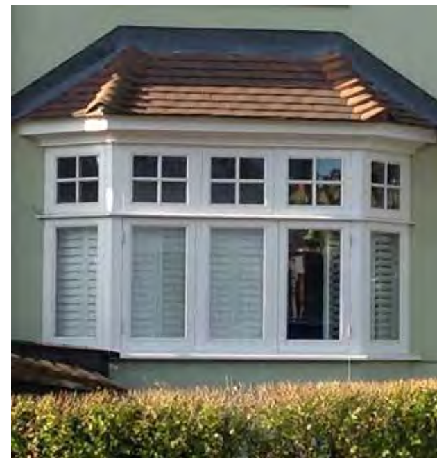
Mid 20th century casement with drip mould
