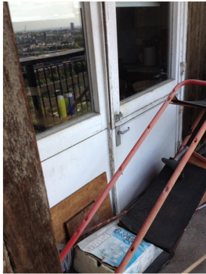
Photo 5 – Kitchen stable door
