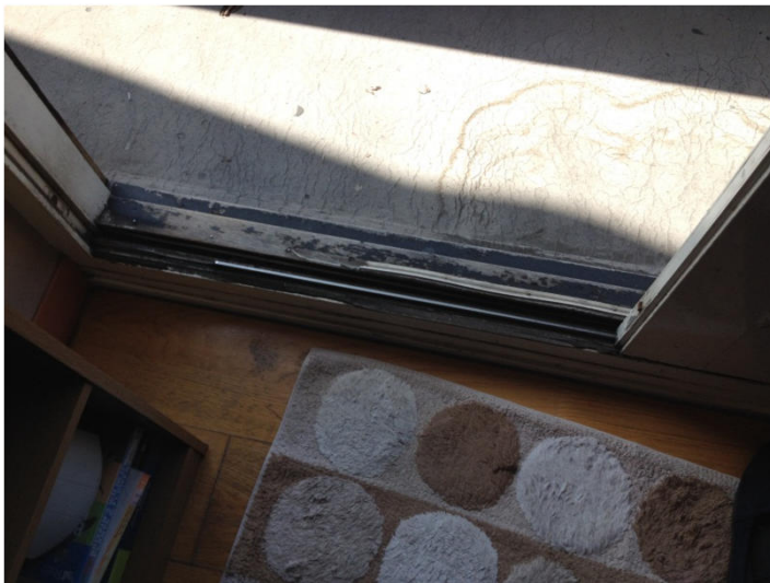
Photo 3 – Sliding balcony door mechanism
