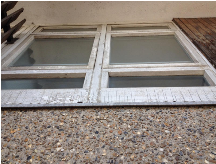
Photo 7 – Upper level window to balcony area
