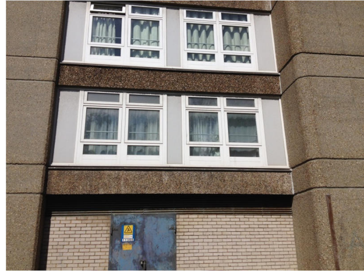
Photo 22 – Replacement window to Block A East Elevation
