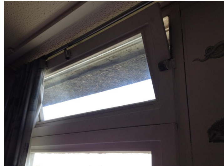
Photo 10 – Centre pivot operating mechanism
