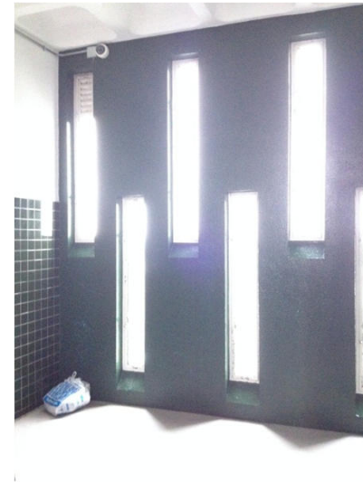
Photo 30 – Service tower window
