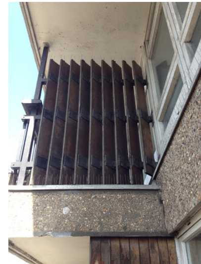
Photo 8 – Balcony timber balustrading
