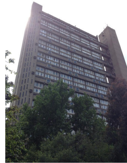
Photo 26 – North elevation of Block A
