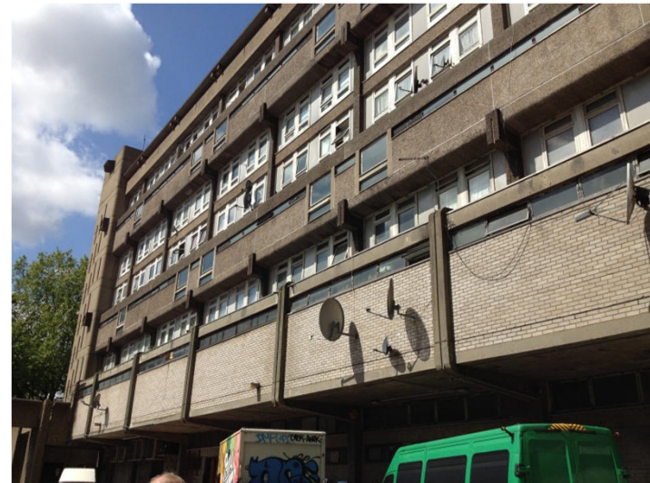
Photo 18 – East Elevation of Block B
