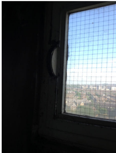
Photo 13 – Georgian wired glass to communal window
