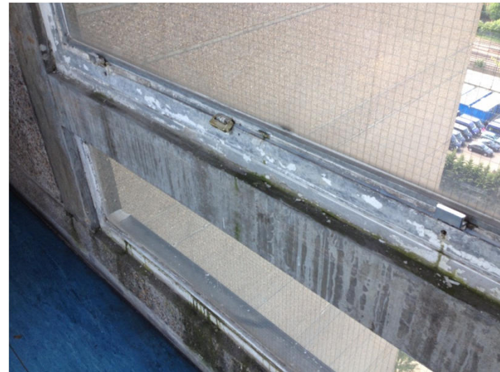
Photo 14 – Internal face of communal window to link bridge
