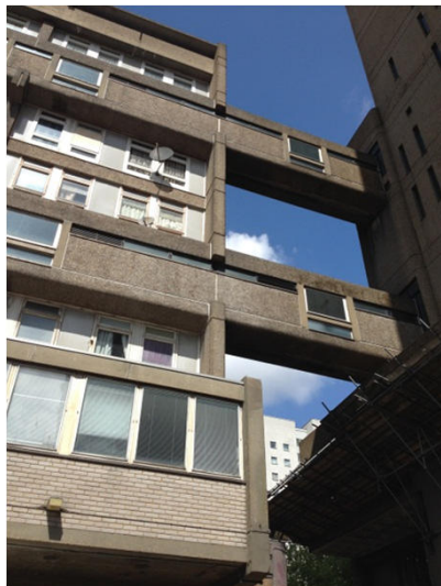
Photo 19 – Links between Block B and service tower
