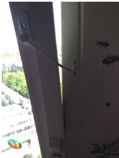
Photo 11 – Jackloc cable restrictor
