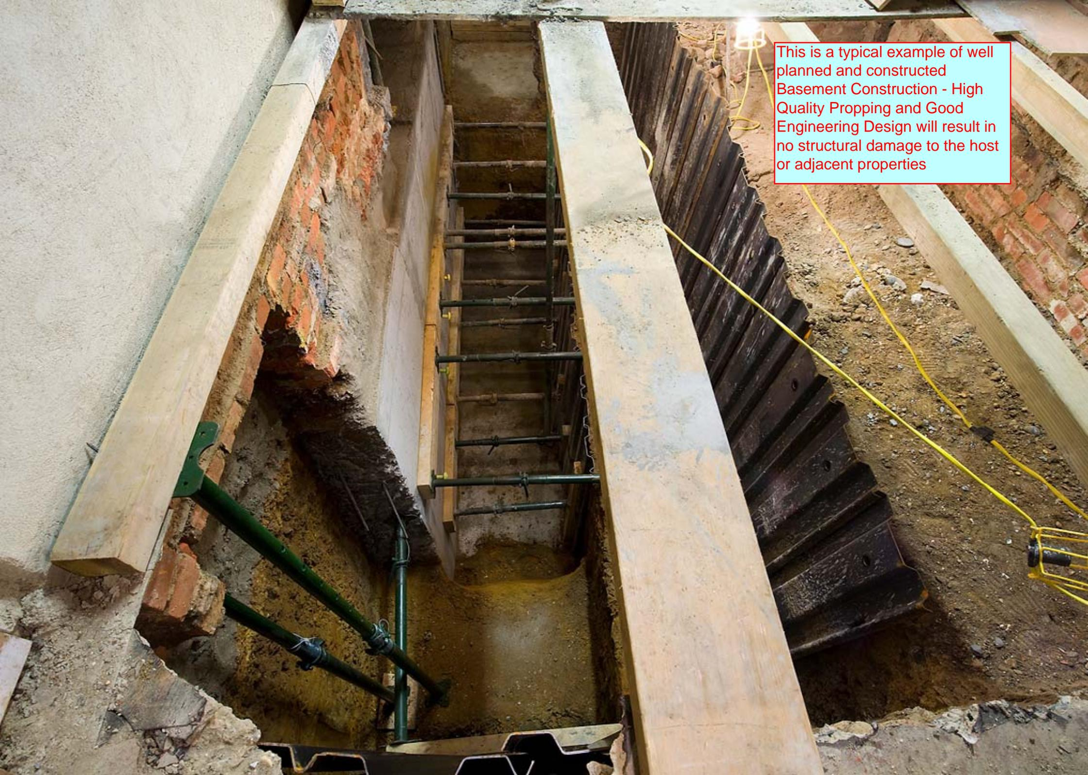
This is a typical example of well planned and constructed Basement Construction - High Quality Propping and Good Engineering Design will result in no structural damage to the host or adjacent properties
