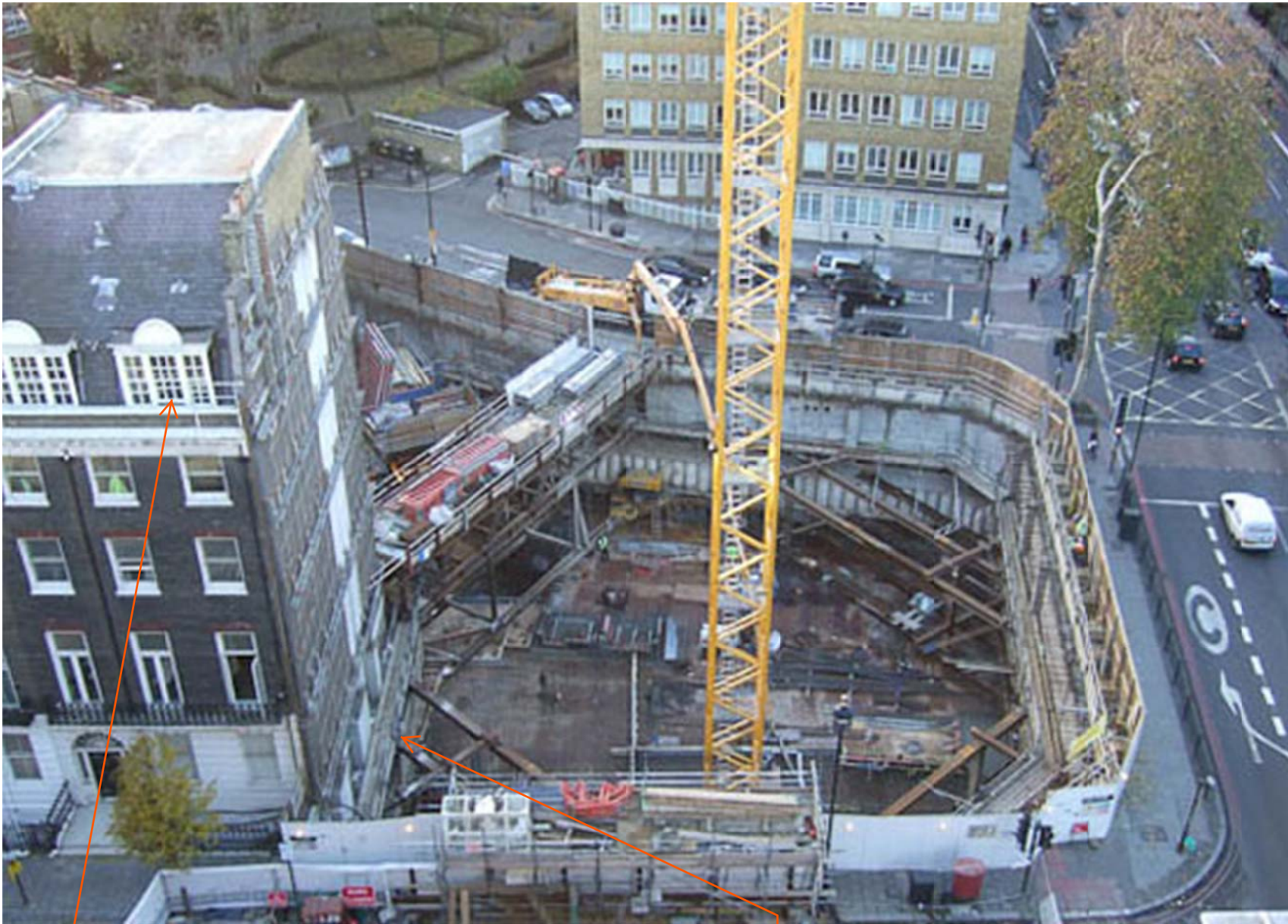
15m Deep Basement - Tight to Flank of Listed Building
