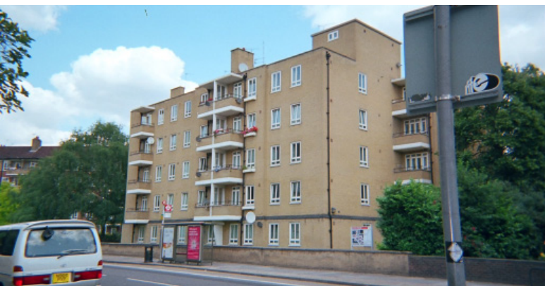
13 Council estates on North End Road north of West Cromwell Road
