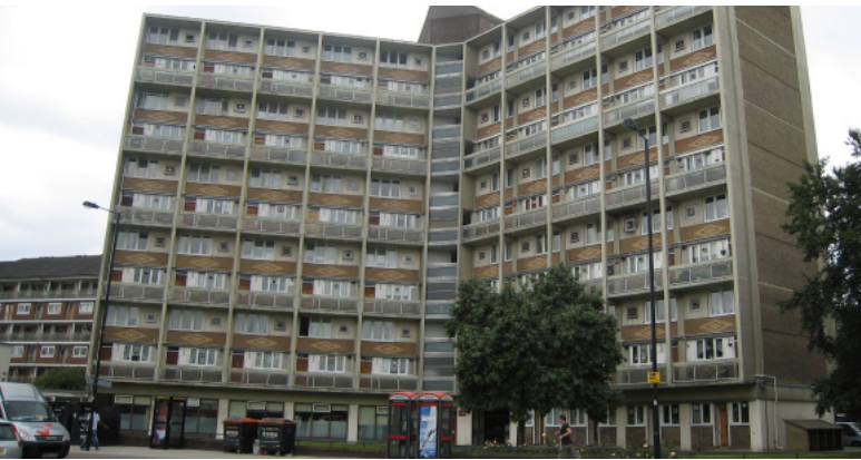
7 Clem Atlee housing estate at Lillie Road / North End Road intersection
