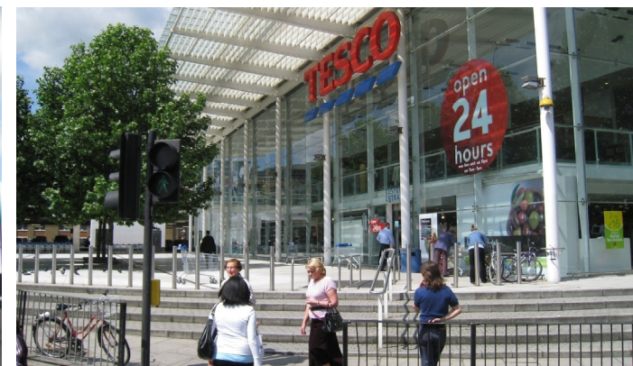
15 Tesco building on the northwest corner of the Warwick Road / A4 West Cromwell Road intersection
