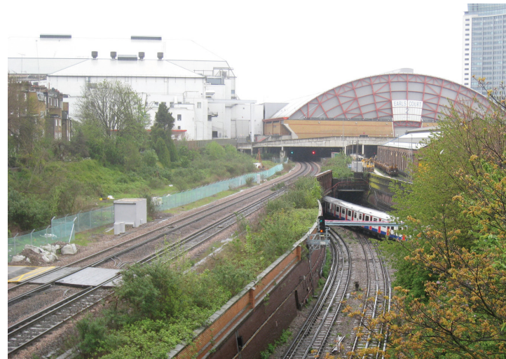
8 Rail lines in the eastern portion of the Regeneration Area
