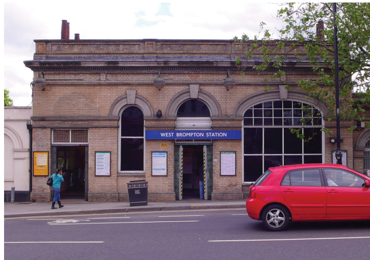
5 West Brompton station
