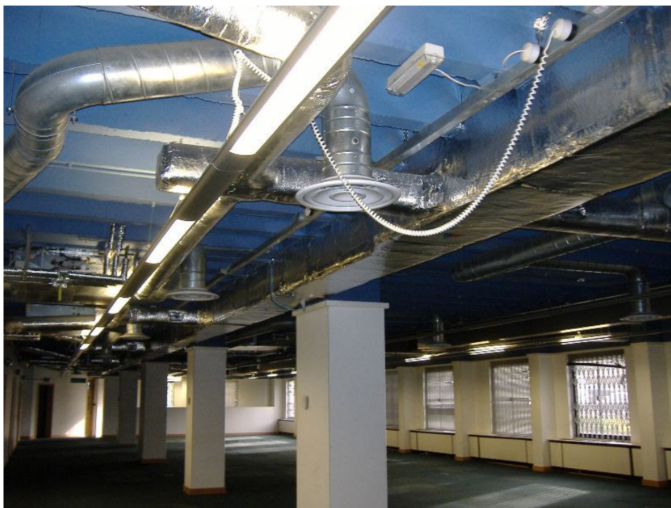
Internal View of Ground Floor
