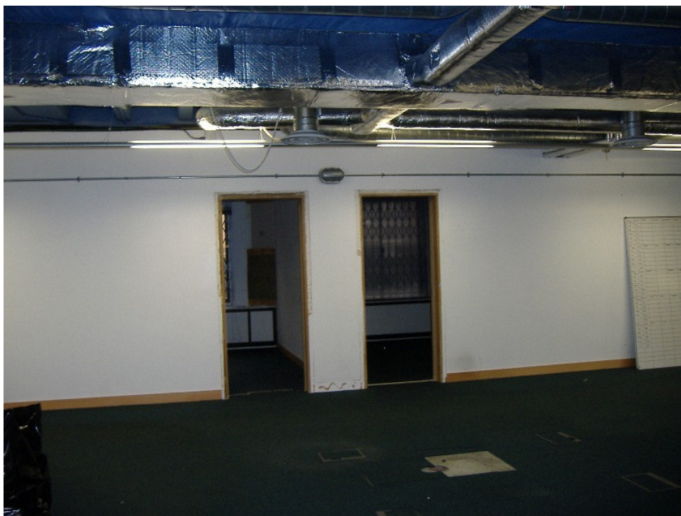
Internal View of Ground Floor
