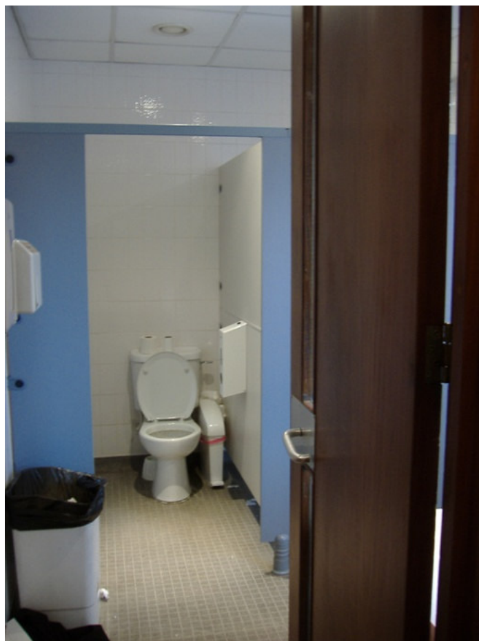
Internal Views of Typical Building Toilet
