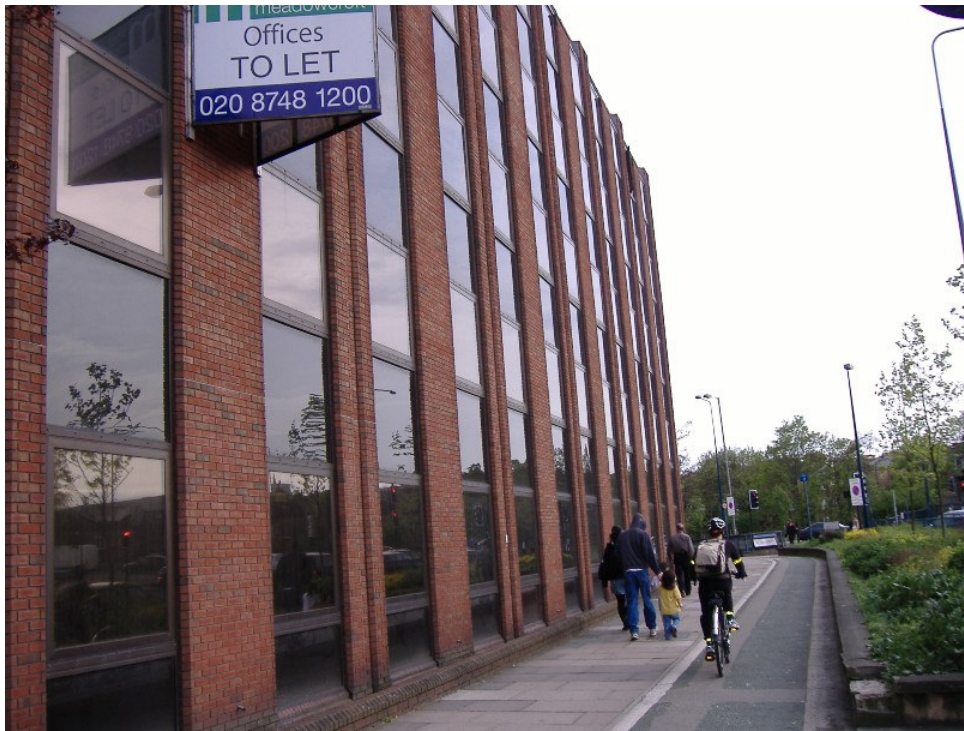
External Elevation Looking West
