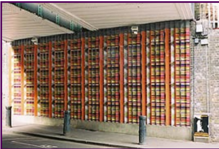
London Underground Railway bridge, Portobello Road (Westway Project)
