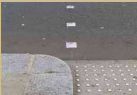
Quadrant kerb with stainless steel tactile paving – Kensington High Street
