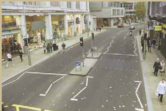
Minimal zig zag markings – Kensington High Street
