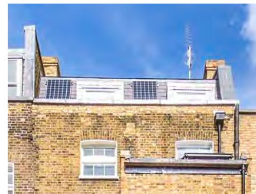
PV installation on a roof (house) over the tiles
