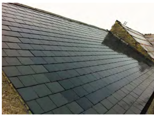
PV installation on a roof (house) – PV slates
