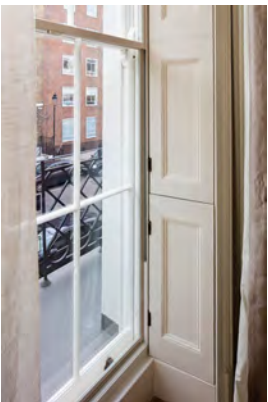
Sliding sash and casement secondary glazing, built into the joinery of the shutter box, within a listed Georgian townhouse.
