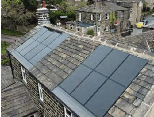
PV installation on a roof (house) as tile replacement
