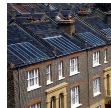
PV installation on a roof (house) over the tiles
