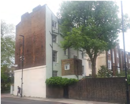
Townhouses within a conservation area in London. Add hoc render has been added to rear facades without disrupting the street scene.
