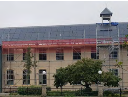
PV installation (rear elevation) over the tiles
