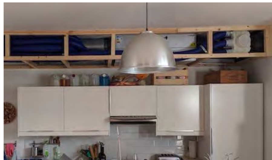
MVHR units can be retrofitted into ceiling voids or wall mounted (© Will South) Ductwork has to be routed to every room. You will need a qualified installer and/or an MVHR manufacturer/supplier to calculate the fresh air required and to design the ventilation system for your home.
