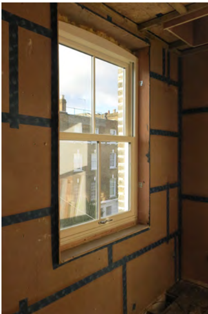
Wood fibre insulation panels fixed and taped with airtightness tape before plasterboard and batten lining
