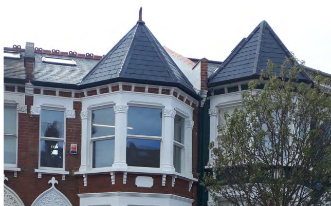
Triple glazed mock sash window
