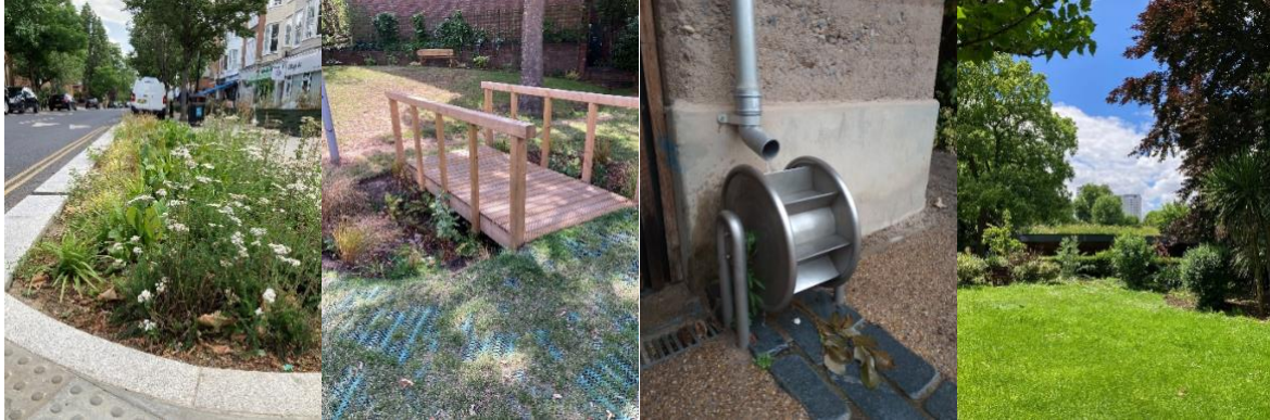
Left to right: rain garden in St Helen's Gardens streetscape improvement scheme, rain garden in Verity Close Green Space improvement scheme, educational downpipe waterwheel on Ecology Centre in Holland Park, green roof on Avondale Park kiosk.
