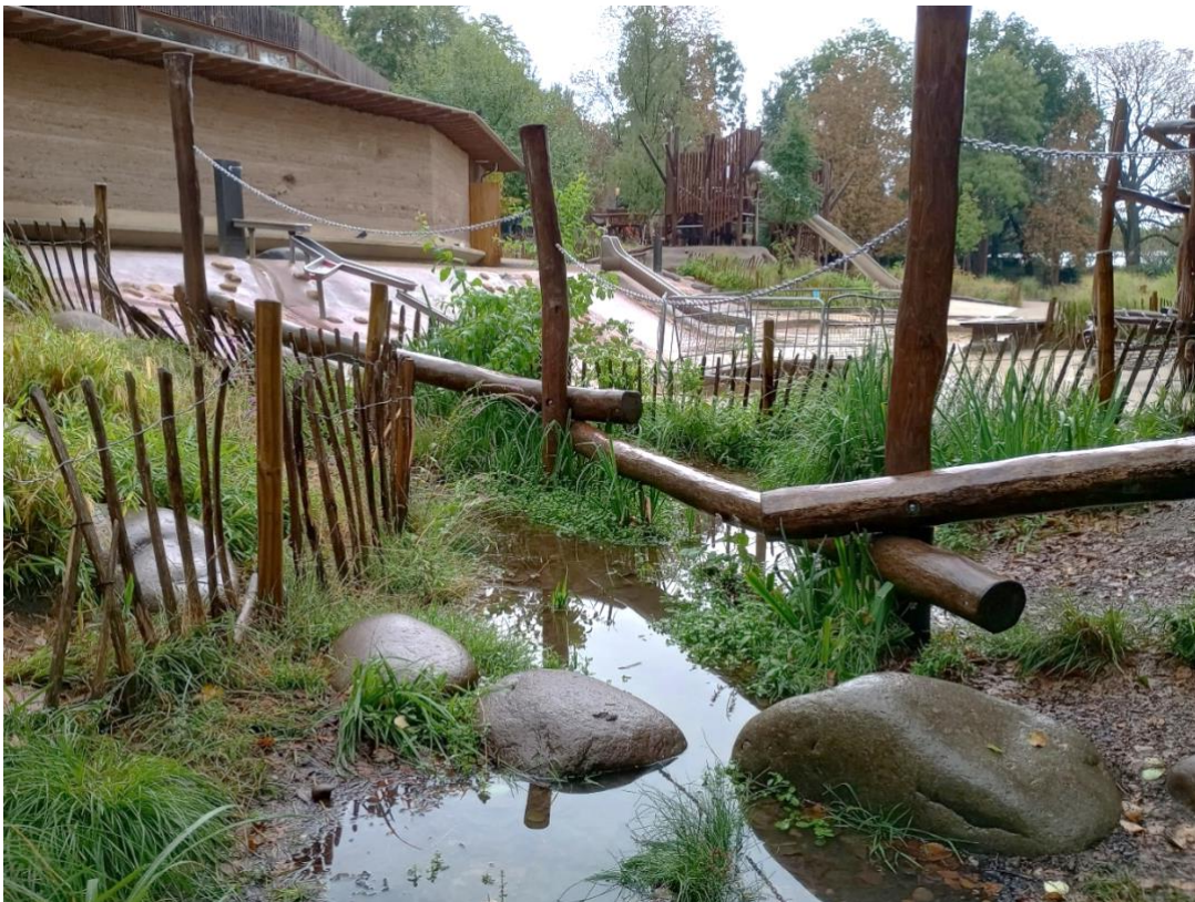
Water flowing through Holland Park Adventure Playground SuDS scheme
