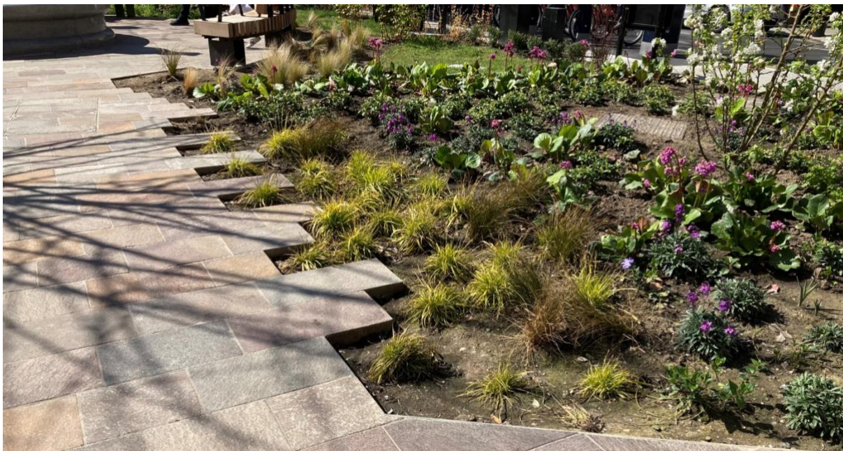
Flush thresholds to planting beds at Chelsea Green streetscape improvement scheme.
