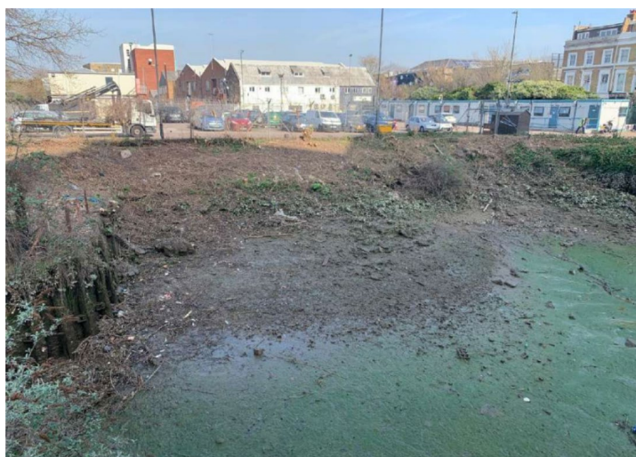
Current condition of the creek wall, with back-filled section between the walled sections clearly visible.
