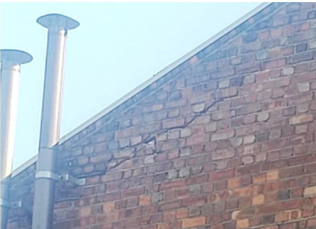
Figure B.6 Cracks in brickwork along the western stretch of the Auction Houses
