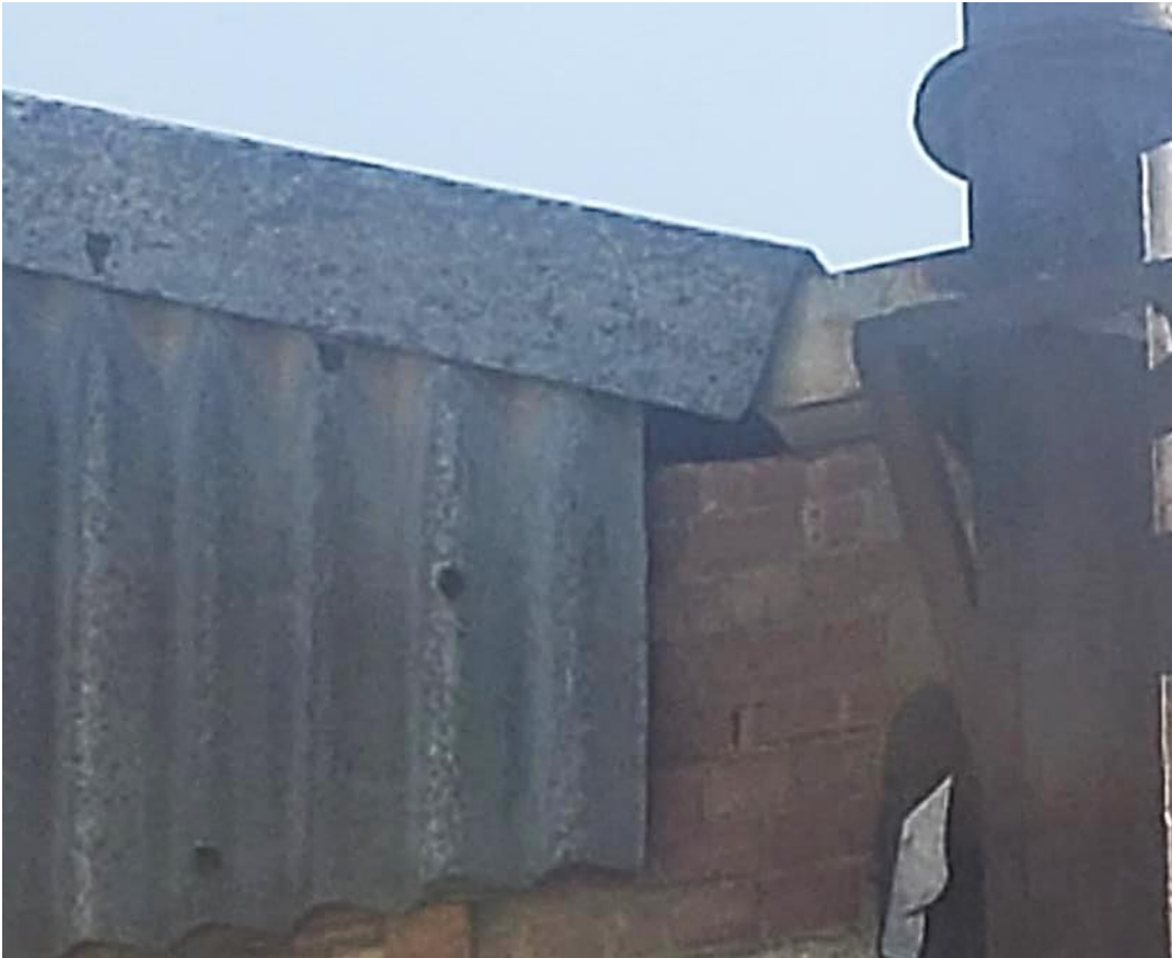
Figure B.7 Gap under lead flashing at the corner of a pitched roof on the southwest side of the Auction Houses
