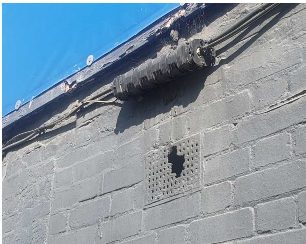
Figure B.4 Broken grate on the south end of the main stretch of buildings along Lots Road
