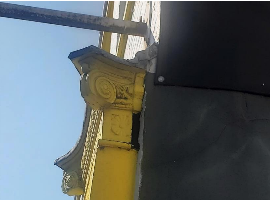
Figure B.8 Soffit hole on the far northeast corner of the Auction Houses along Lots Road
