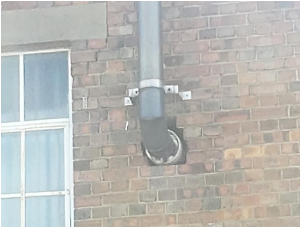
Figure B.5 Gaps between brickwork and pipe along the western stretch of the auction houses - there are several of these
