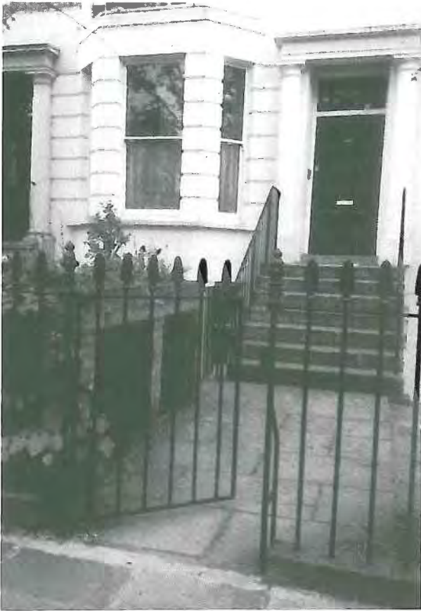
Modern railings which work well and better binstores
