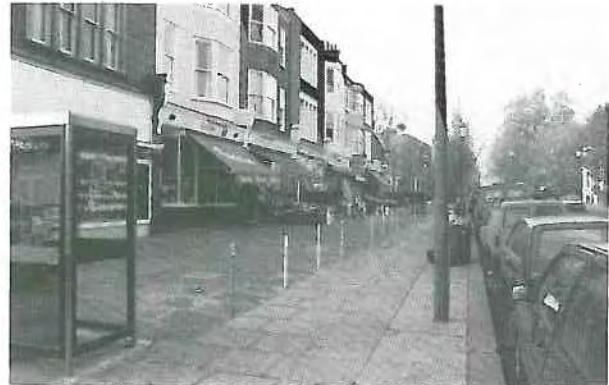
Unsatisfactory demarcation of the shopping parade
