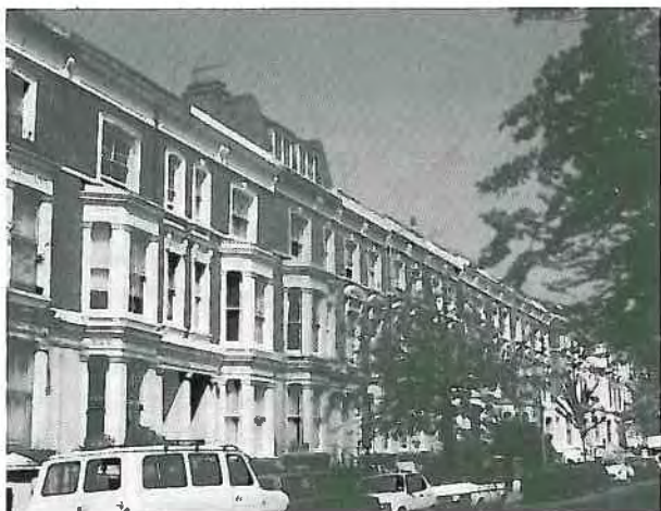
This isolated roof addition in Chesterton Road does not set a precedent
