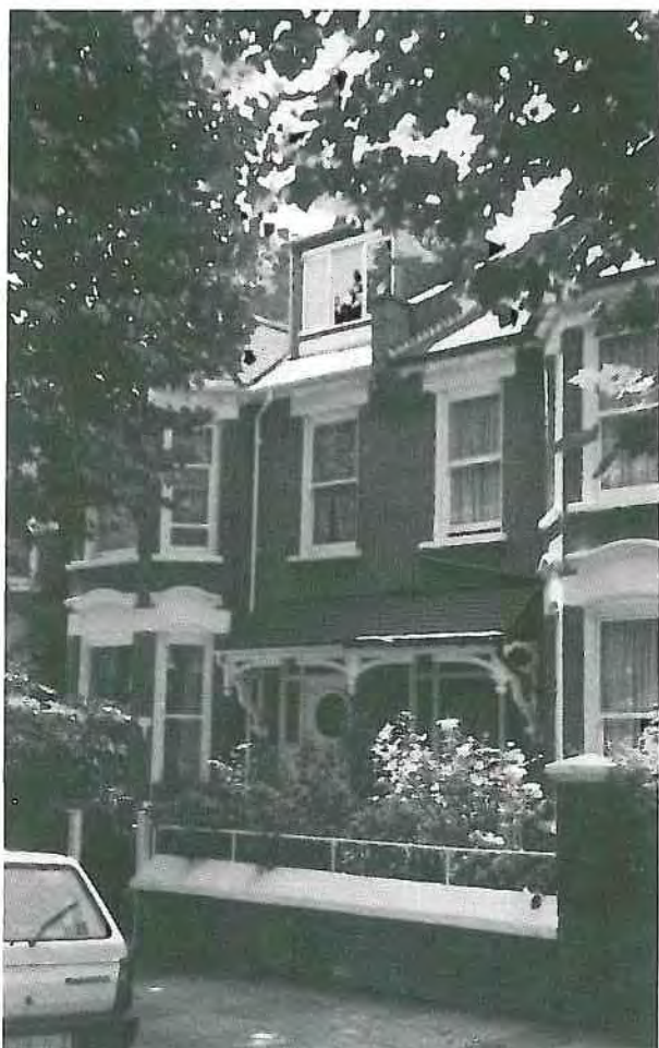
Dormer as extra storey in Highlever Road
