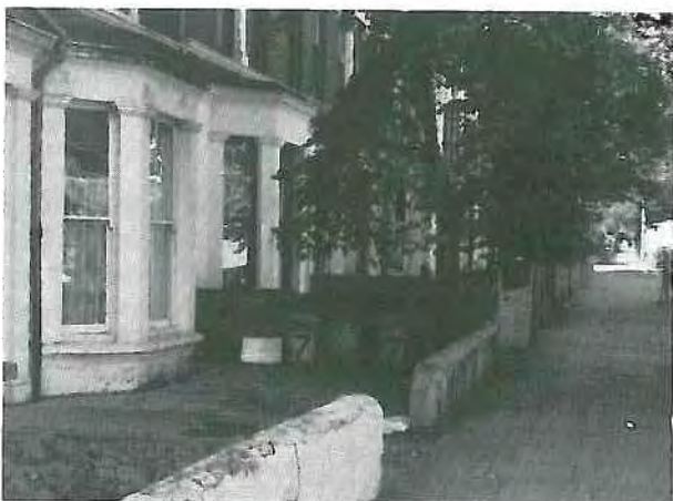
Weak boundary treatment and no binstores
