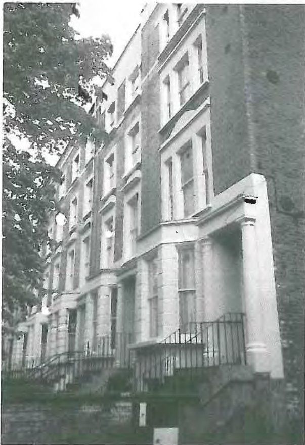
Attentive repair rather than restoration in Oxford Gardens
