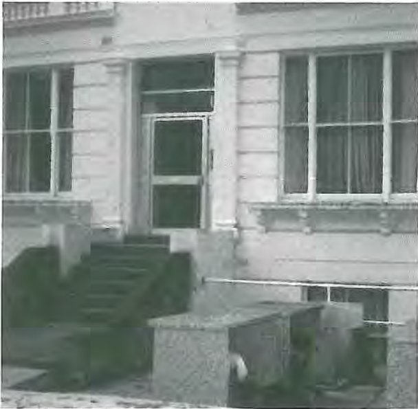
...and ill-considered binstores
