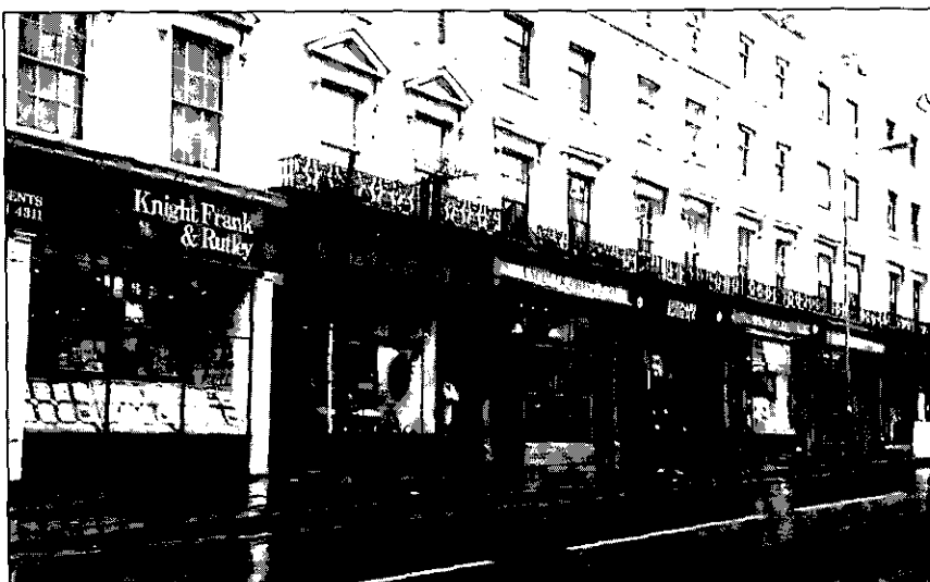
“Category A” shopfronts at 67-81 Kensington Church Street
