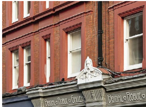
Façade articulation in contemporary and local buildings
