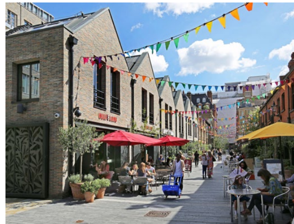
Paving material extending to building façade
